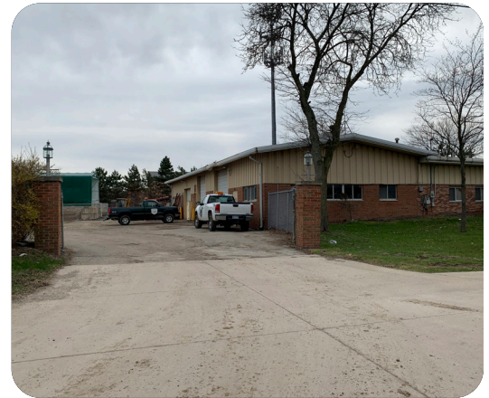
Lathrup Village DPS yard (Giffels Webster, 2020)
