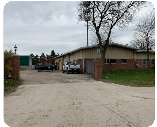
Lathrup Village DPS yard (Giffels Webster, 2020)
