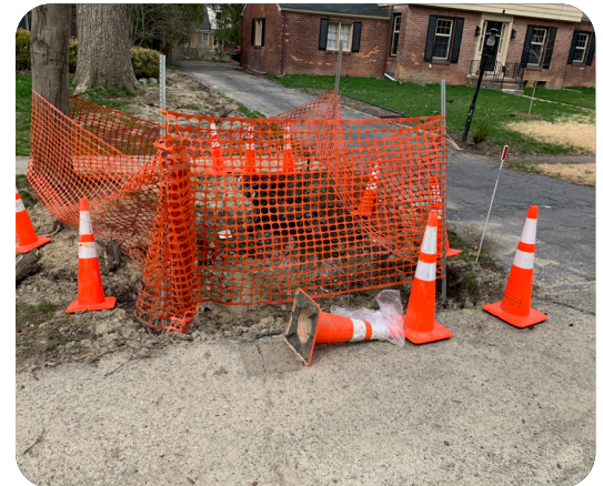
Drainage ditch repair (Giffels Webster, 2020)
