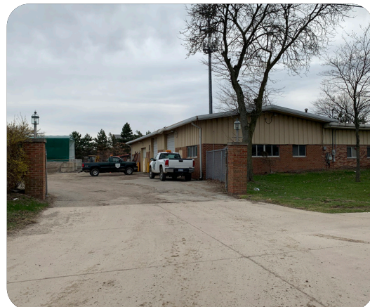
Lathrup Village DPS yard (Giffels Webster, 2020)
