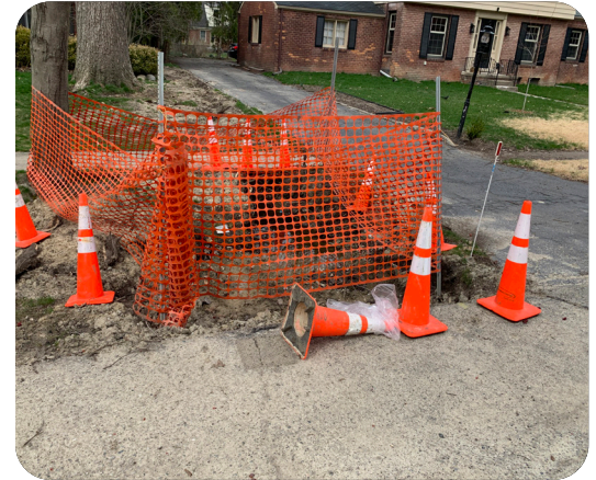
Drainage ditch repair (Giffels Webster)
