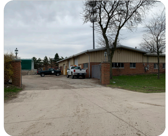
Lathrup Village DPS yard (Giffels Webster)
