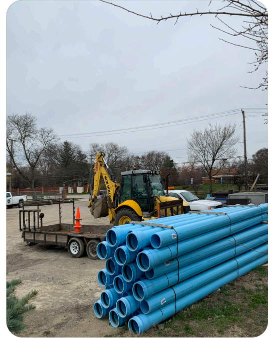
Lathrup Village DPS yard (Giffels Webster, 2020)
