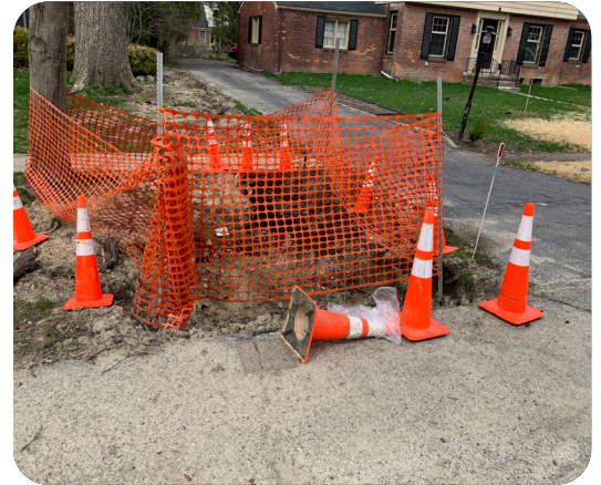
Drainage ditch repair (Giffels Webster, 2020)
