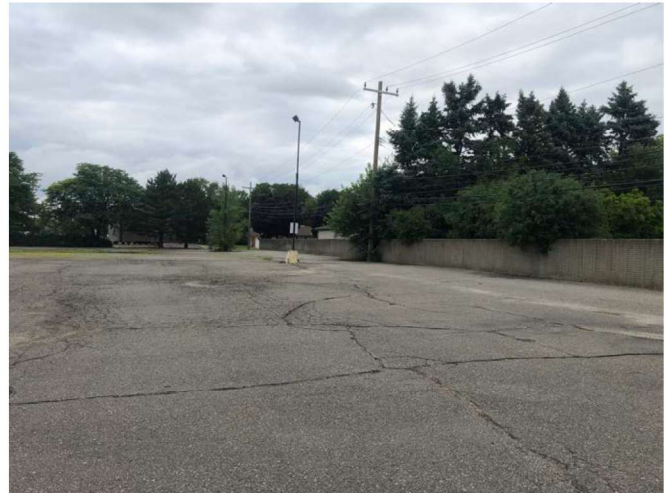
Above: 26026 Southfield Road abuts single family homes and is separated by an existing masonry wall.
