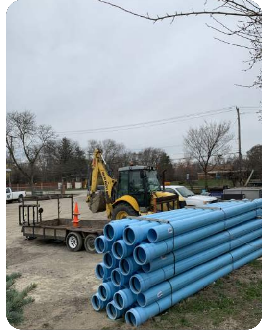
Lathrup Village DPS yard (Giffels Webster, 2020)
