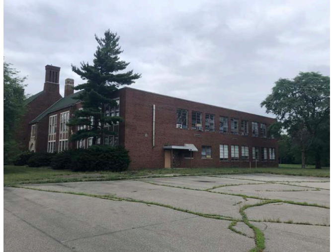
Above: The Annie Lathrup School site is vacant with large adjacent parking lots.
