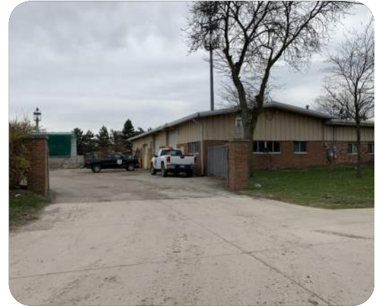
Lathrup Village DPS yard (Giffels Webster, 2020)
