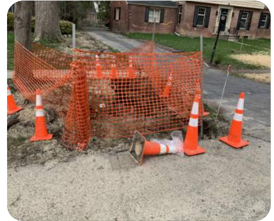
Drainage ditch repair (Giffels Webster, 2020)
