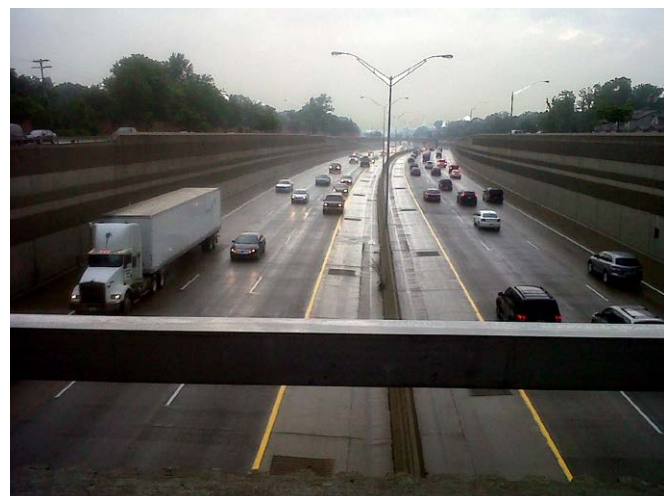
I-696 through Lathrup Village
