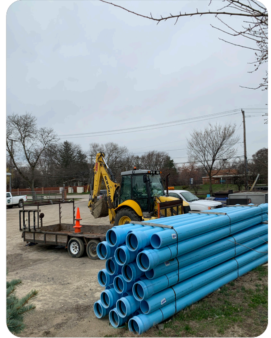
Lathrup Village DPS yard (Giffels Webster, 2020)
