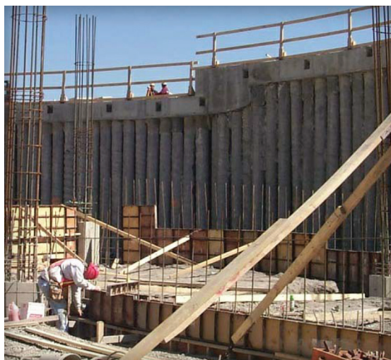
Earth Retention Wall Design and Construction
