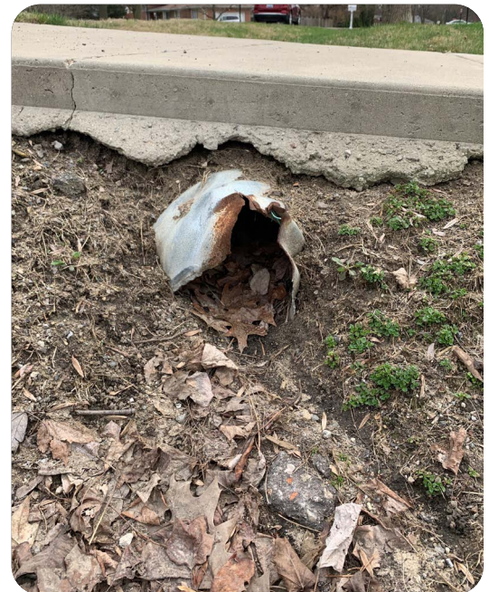
Damaged storm sewer culvert (Giffels Webster, 2020)
