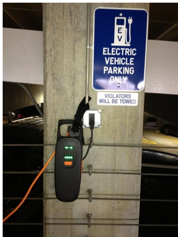
Photo 6. One of many highly visible Level 1 charging stations at Coca-Cola. The driver straps the cordset to the electrical conduit so there is no strain on the plug and outlet. The parking spot is well marked with an Electric Vehicle Parking Only sign.
