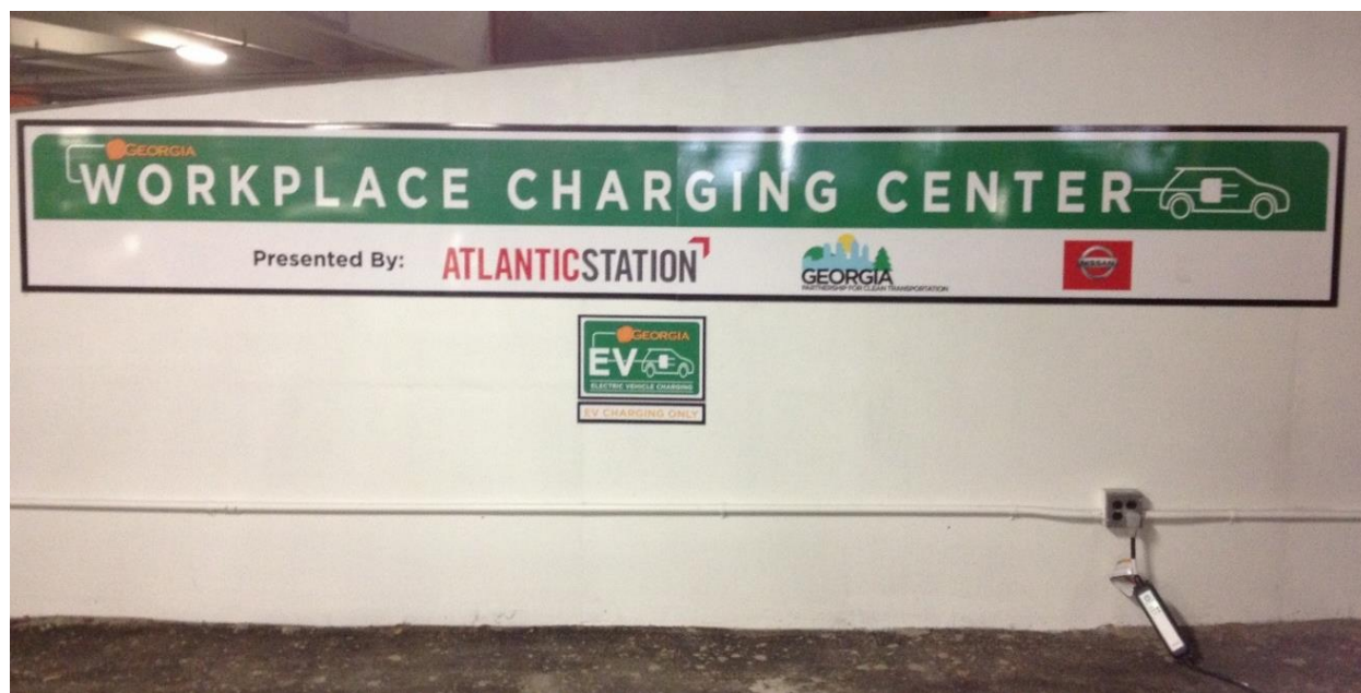
Photo 12. Atlantic Station offers ten Level 1 outlets in a parking garage underneath one of their office towers. These spaces are reserved for the office workers in the building.
