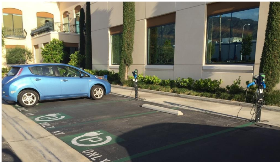
Photo 9. At AeroVironment's Monrovia office, they offer workplace charging using TurboDocks which can be used for Level 1 or Level 2 charging.
