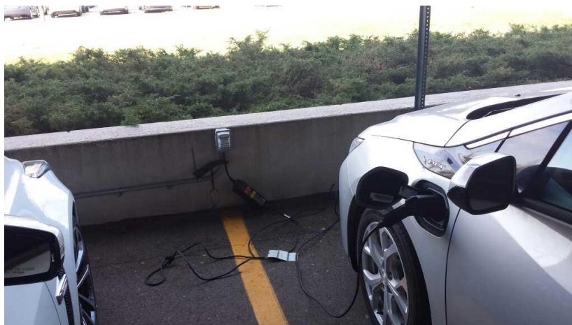
Photo 3. Over 150 Level 1 outlets are available for workplace charging at GM worksites.
