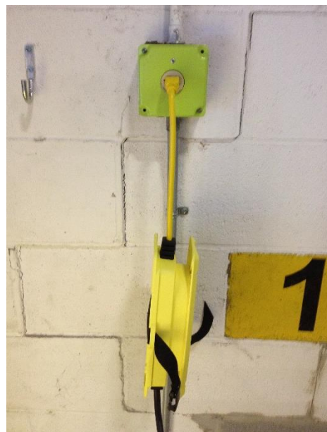
Photo 4. This cordset is hanging from an outlet which may cause strain on the cordset and outlet.
