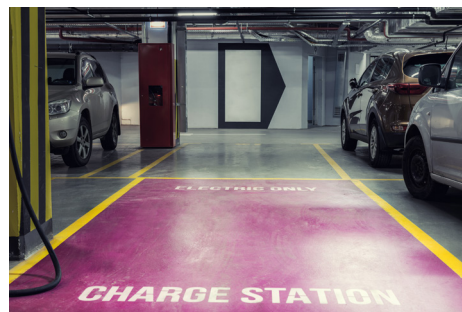
Multi-Family Dwelling Charging
