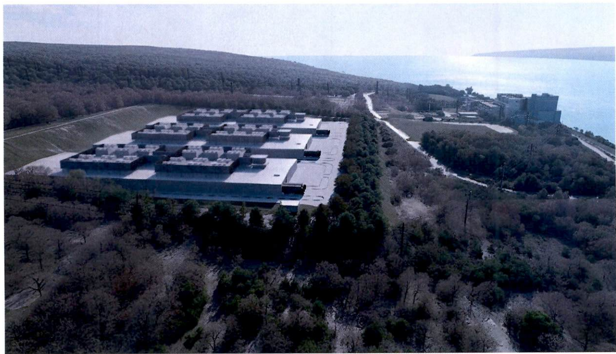
Aerial view — after stack removal.
