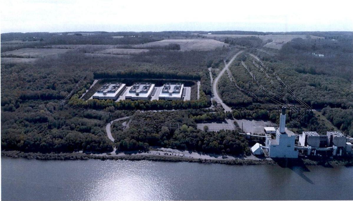
Lakeside aerial view — with former stack.
