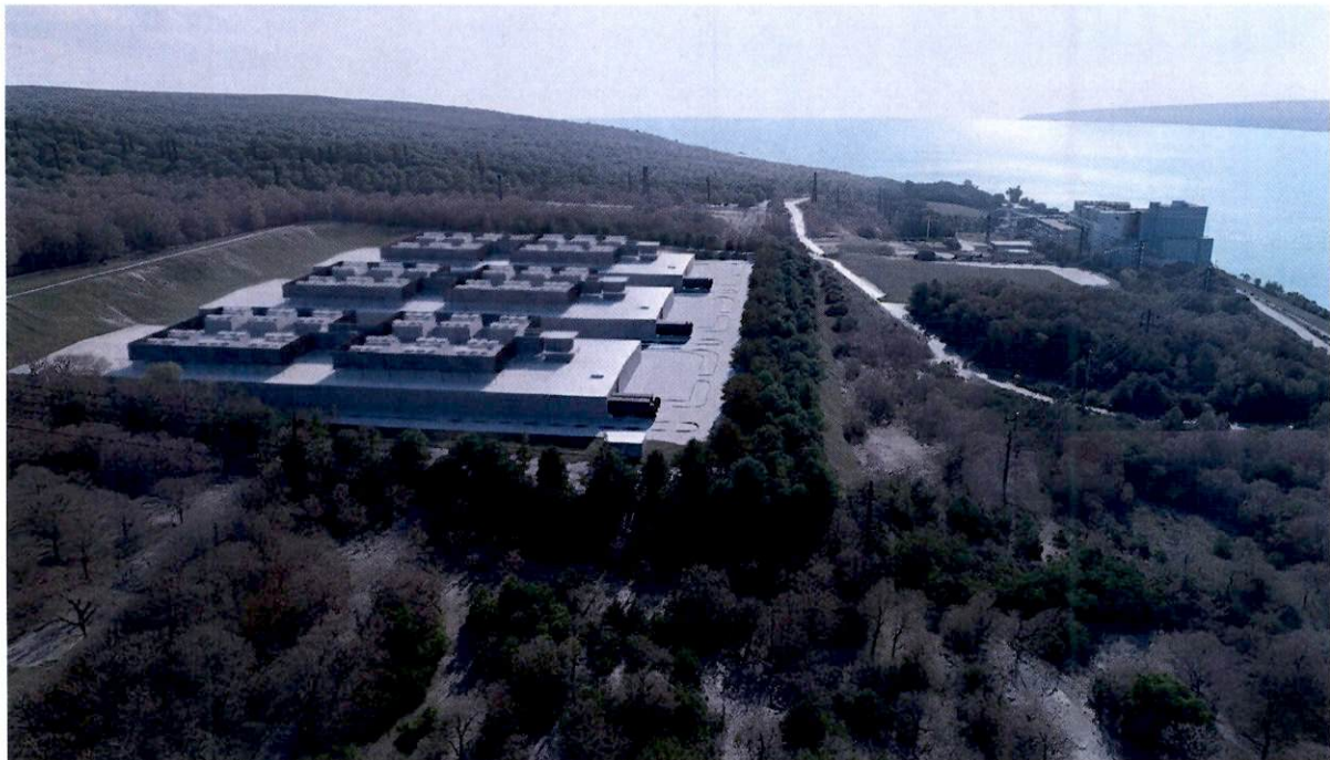
Aerial view — after stack removal.
