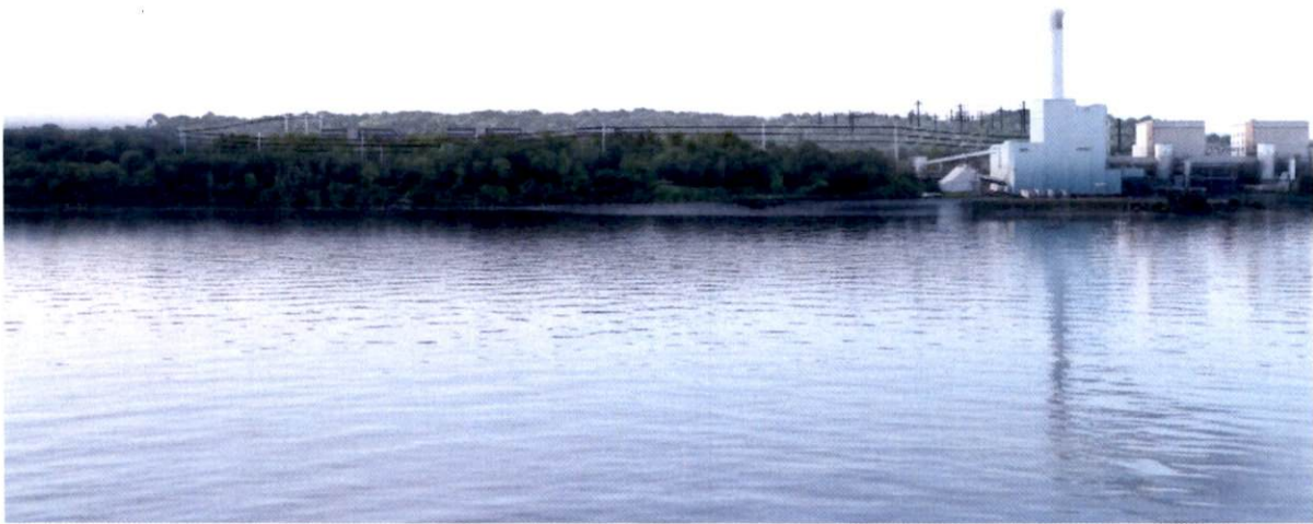
Lakeside ground-level view — with former stack.
