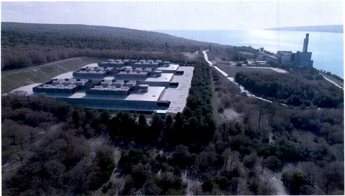
Aerial view — with former stack.
