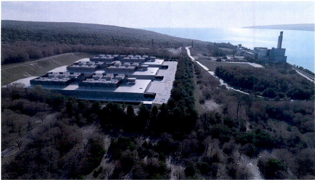
Aerial view — with former stack.
