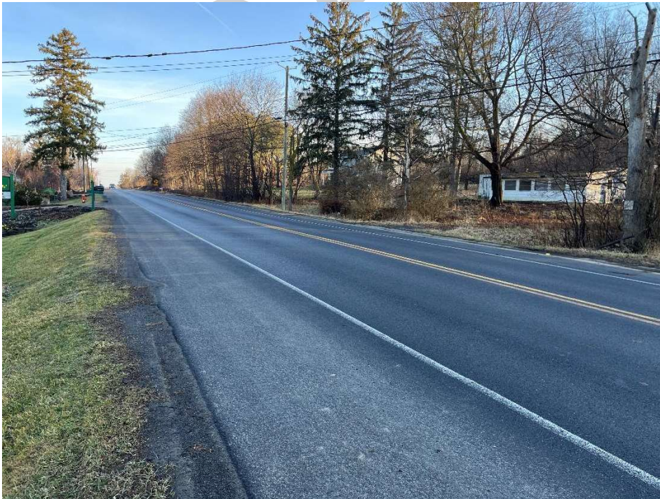
Photo 15 – View of N Triphammer Road, view to the north.
