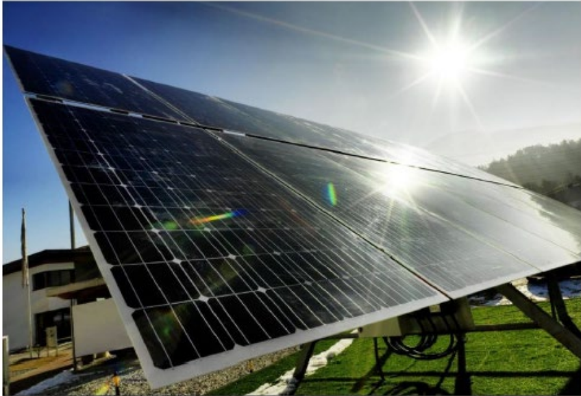
Solar panel showing solar glare
