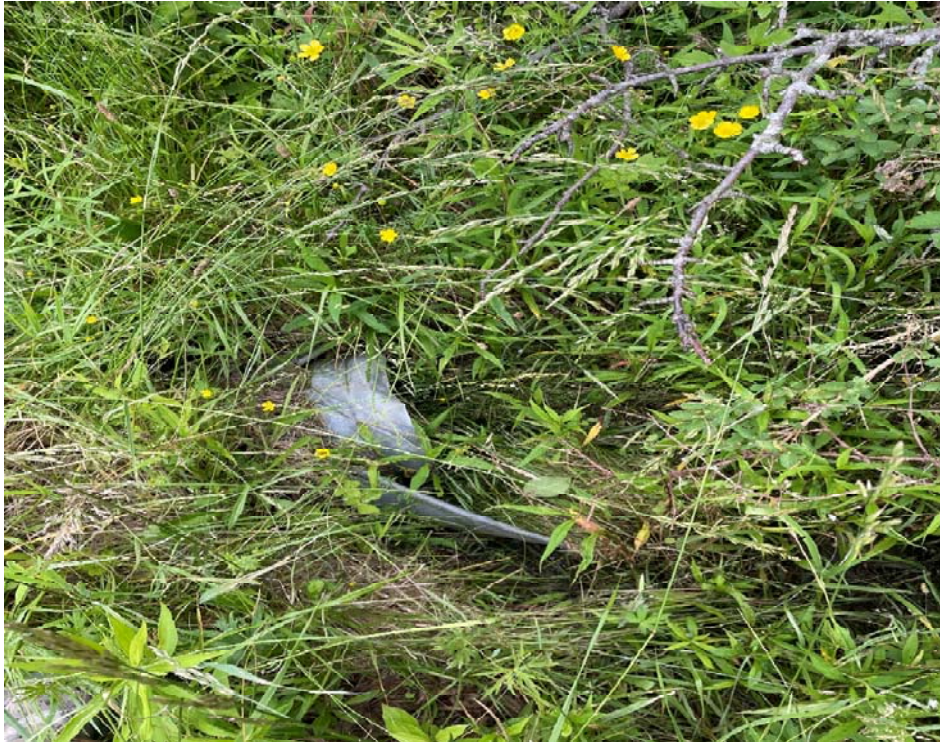
Photo 12. View looking at a pipe culvert feeding water from the 'A/B' flagged wetland towards the 'C/D' wetland.
