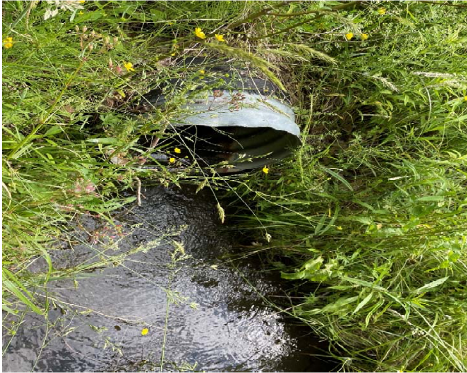
Photo 7. View of a culvert feeding wetland areas within hedgerows .
