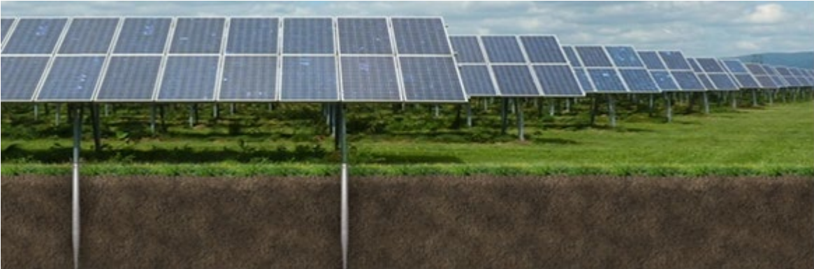
Figure 3b. Supporting Structure Overview
