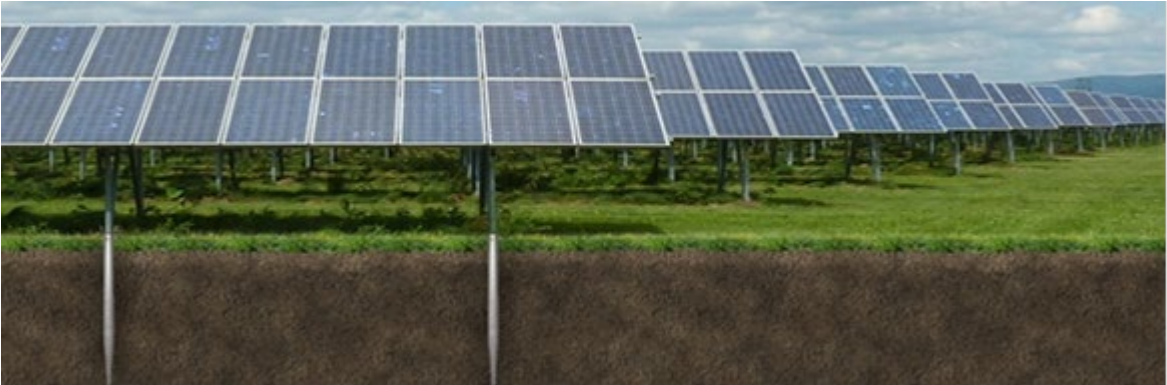
Figure 3b. Supporting Structure Overview
