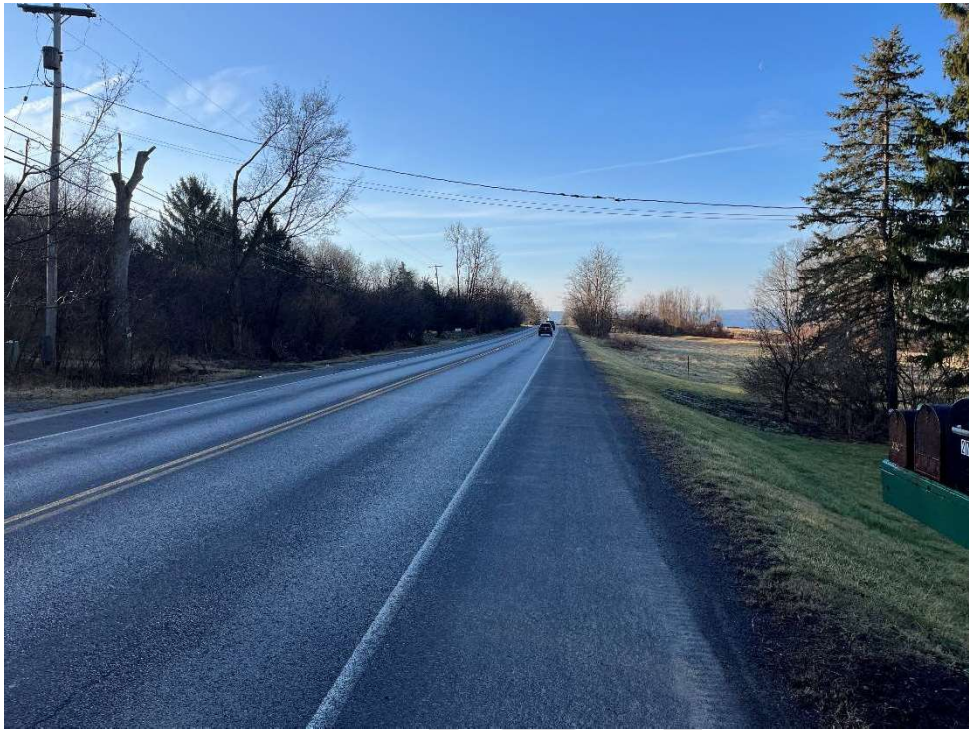
Photo 14- View of N Triphammer road, view to the south.
