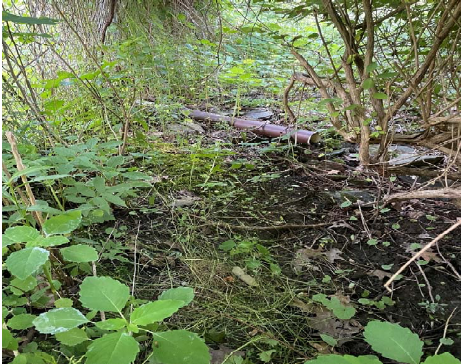
Photo 10. View facing east looking at a pipe culvert feeding water into the site from the northern boundary of the inspection area.
