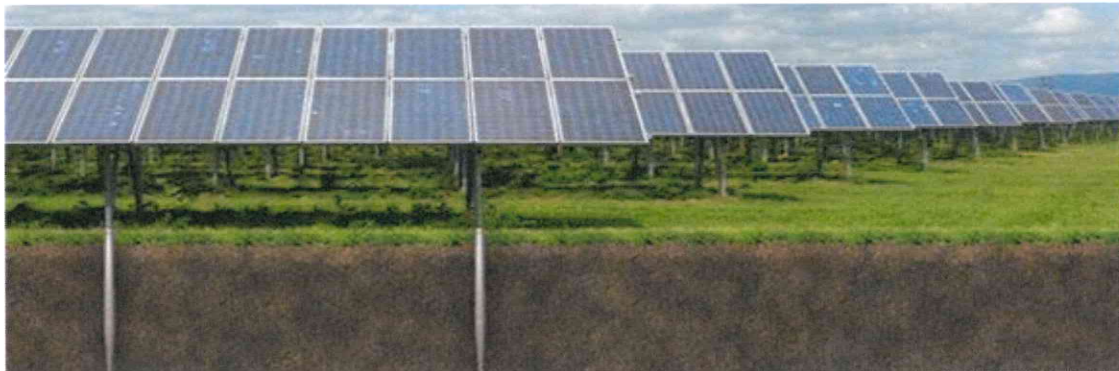
Figure 3b. Supporting Structure Overview
