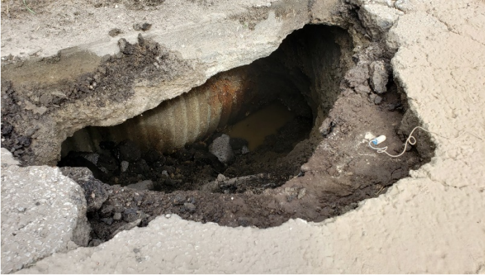
Photo 1(5/28/21) – Valley drive at C.I. – hole in pavement Void area beneath pavement and curb.
