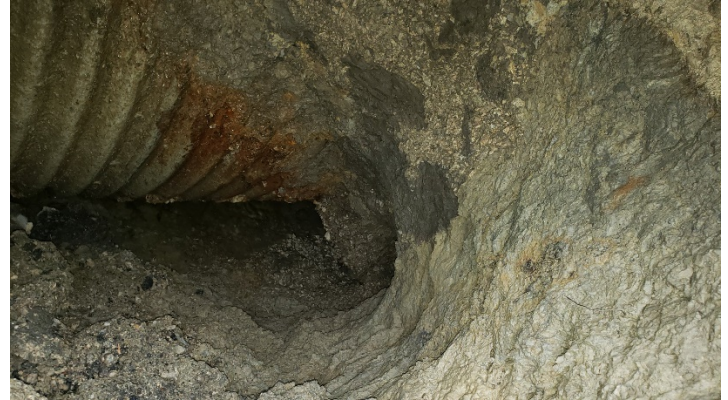
Photo 2 (5/28/21)– Valley Drive downstream of C.I. Rusted out pipe bottom had created a void under the pipe.
