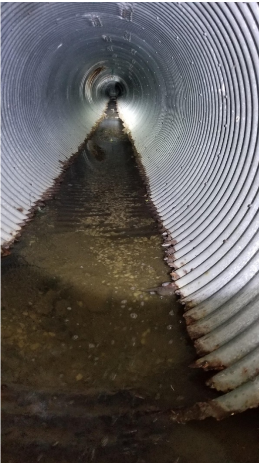
Photo #3 (5/28/21) – Looking down stream from The curb inlet. NOTE: bottom of pipe is completely Rusted the entire length.
