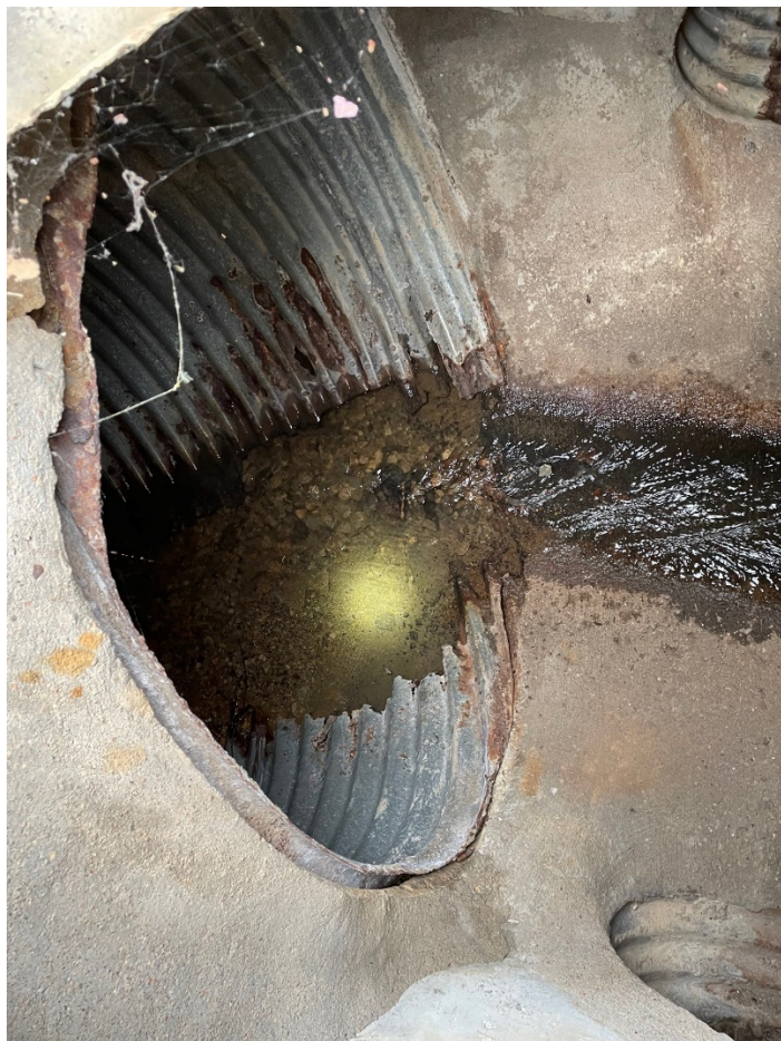
Photo #4 (7/7/21) – Junction box on Valley north of 4H looking downstream NOTE: bottom is rusted out under 4H road as well.
