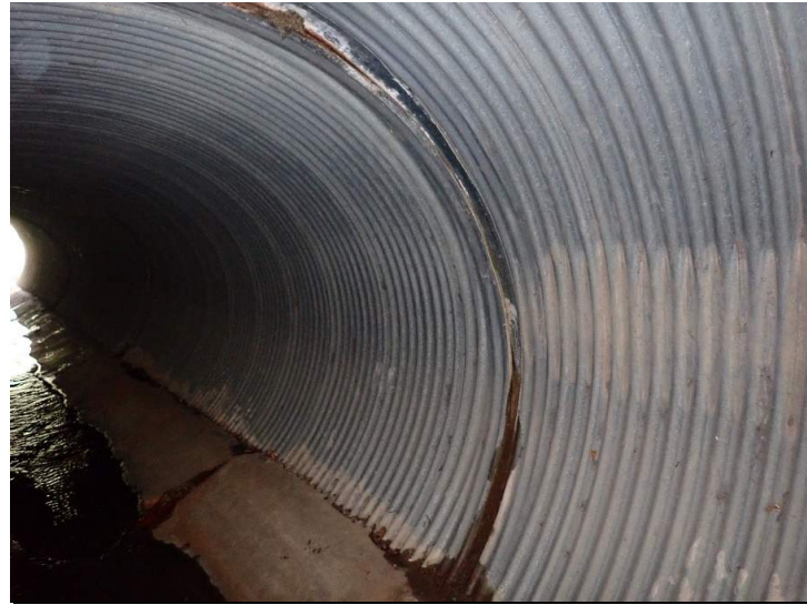
EAST SEAM WITH MINOR LEAKAGE AT NORTH SIDE
