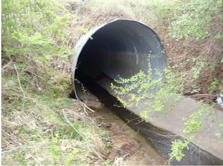
WEST ELEVATION, INLET, NO VISIBLE DEFLECTION
