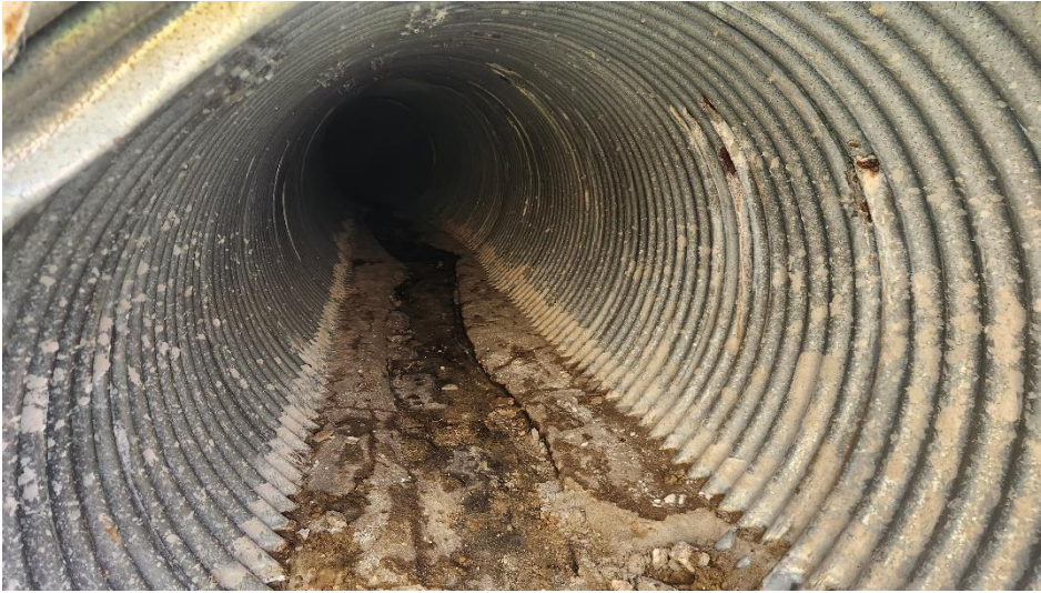
Photo #1 – Existing CMP Pipe under 4H Road
