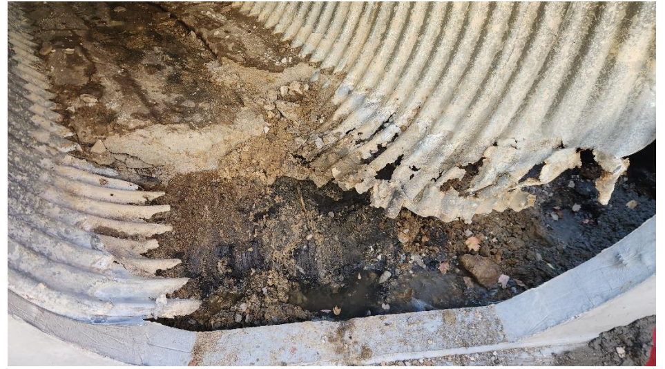
Photo #2 – Interface between new box and existing CMP Pipe
