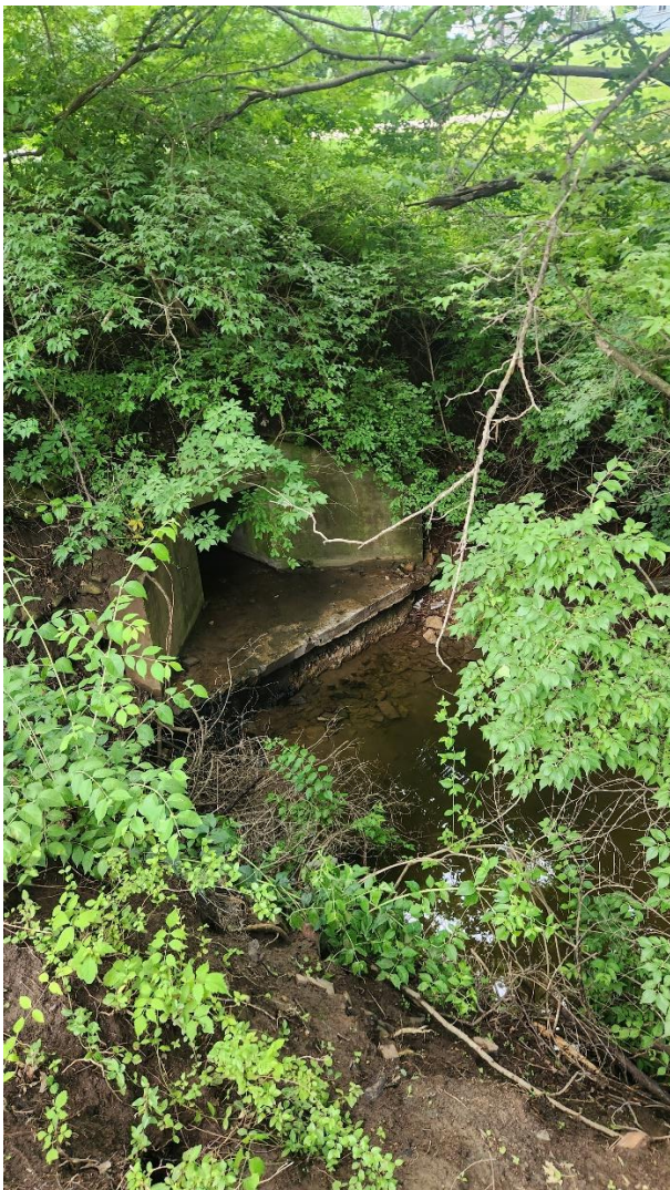
Plunge Pool at Box Culvert Outfall
