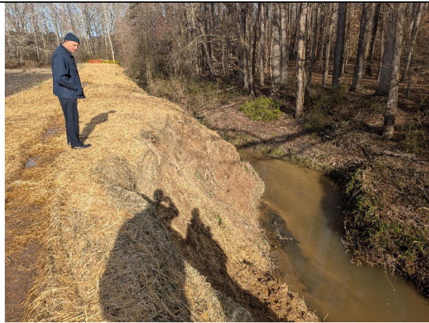
North embankment crest. View looking downstream. Note near-vertical scarp and undermining of crest.
