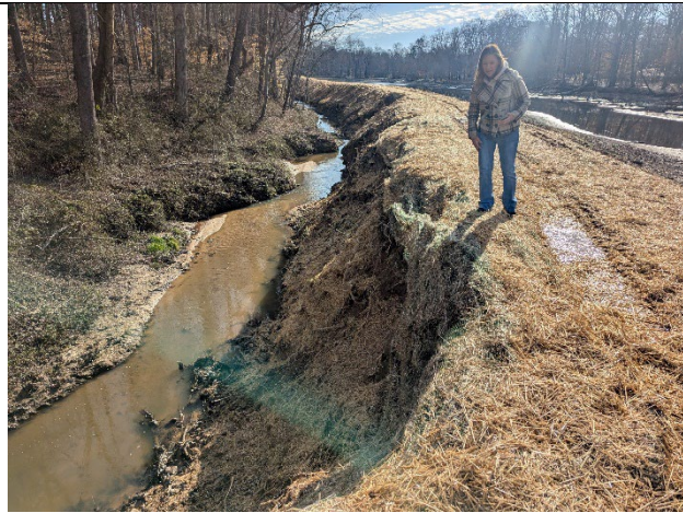
North embankment crest. View looking downstream. Note near-vertical scarp and undermining of crest.
