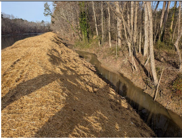
North embankment. View looking upstream along crest. Note standing water and ruts.
