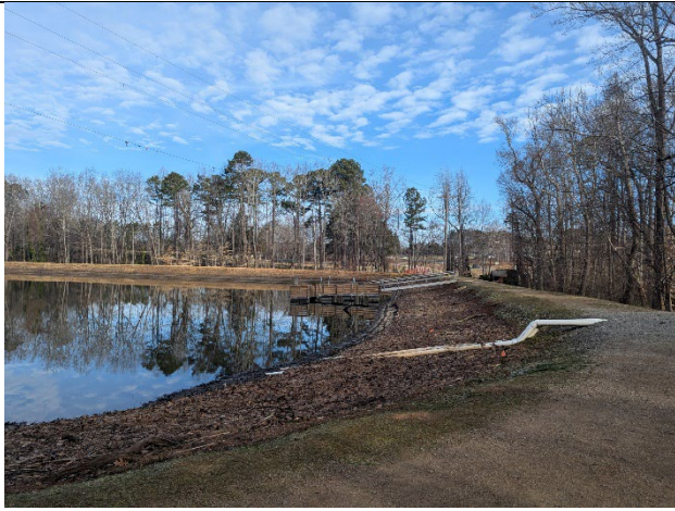
North embankment. View looking upstream along outboard slope. Note seed and straw on slope.
