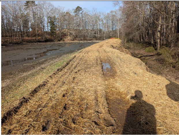
North embankment. View looking upstream along crest. Note standing water and ruts.
