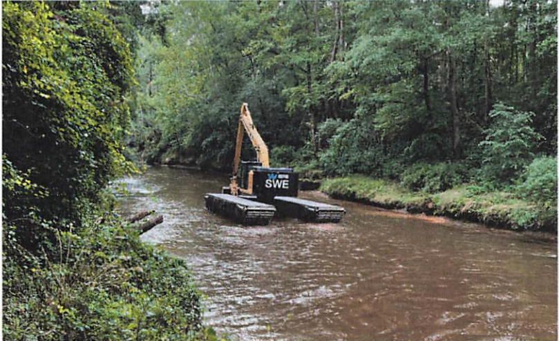
Before & After: Back Swamp Stream Debris Removal
