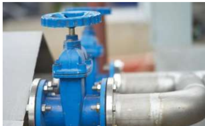
Gate Valve Installation for Isolation $5,000,000
