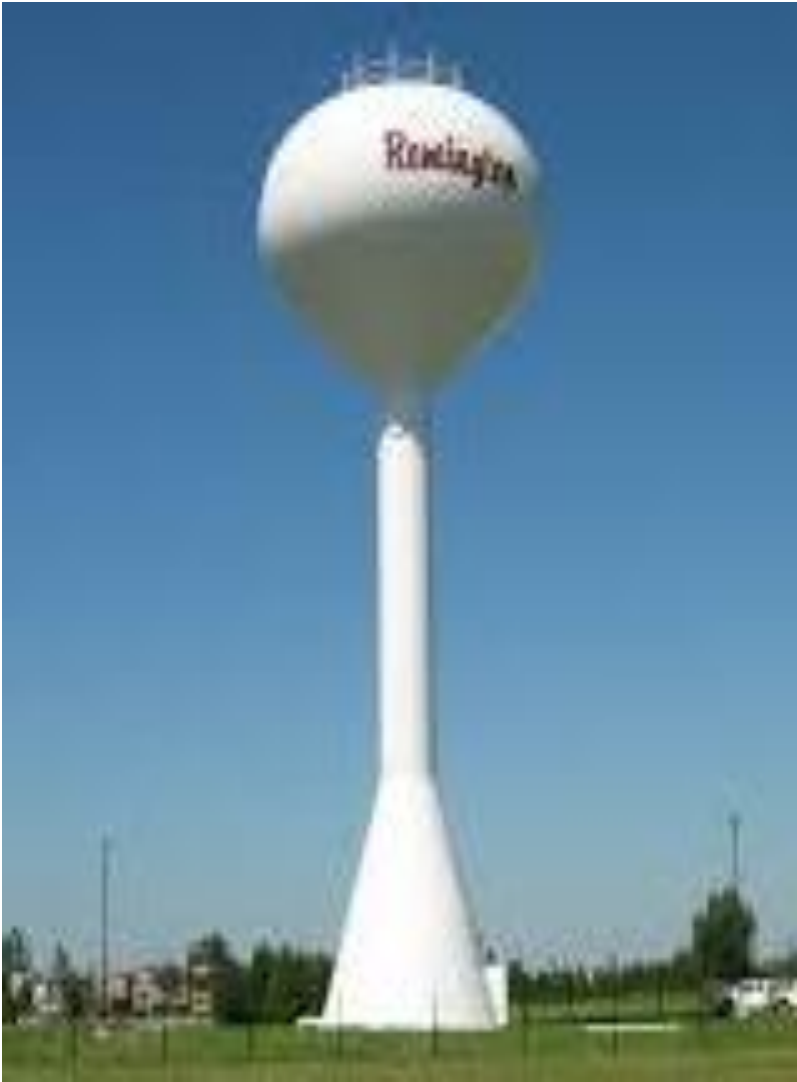
SPHERIOD 100,000 GALLON WATER TANK
