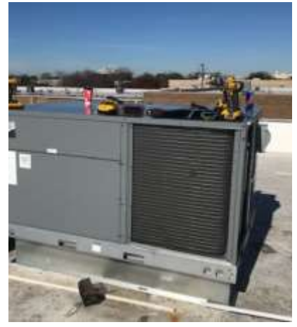
Replace HVAC Unit
