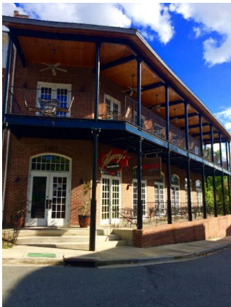
Commercial center (Vermillion)
