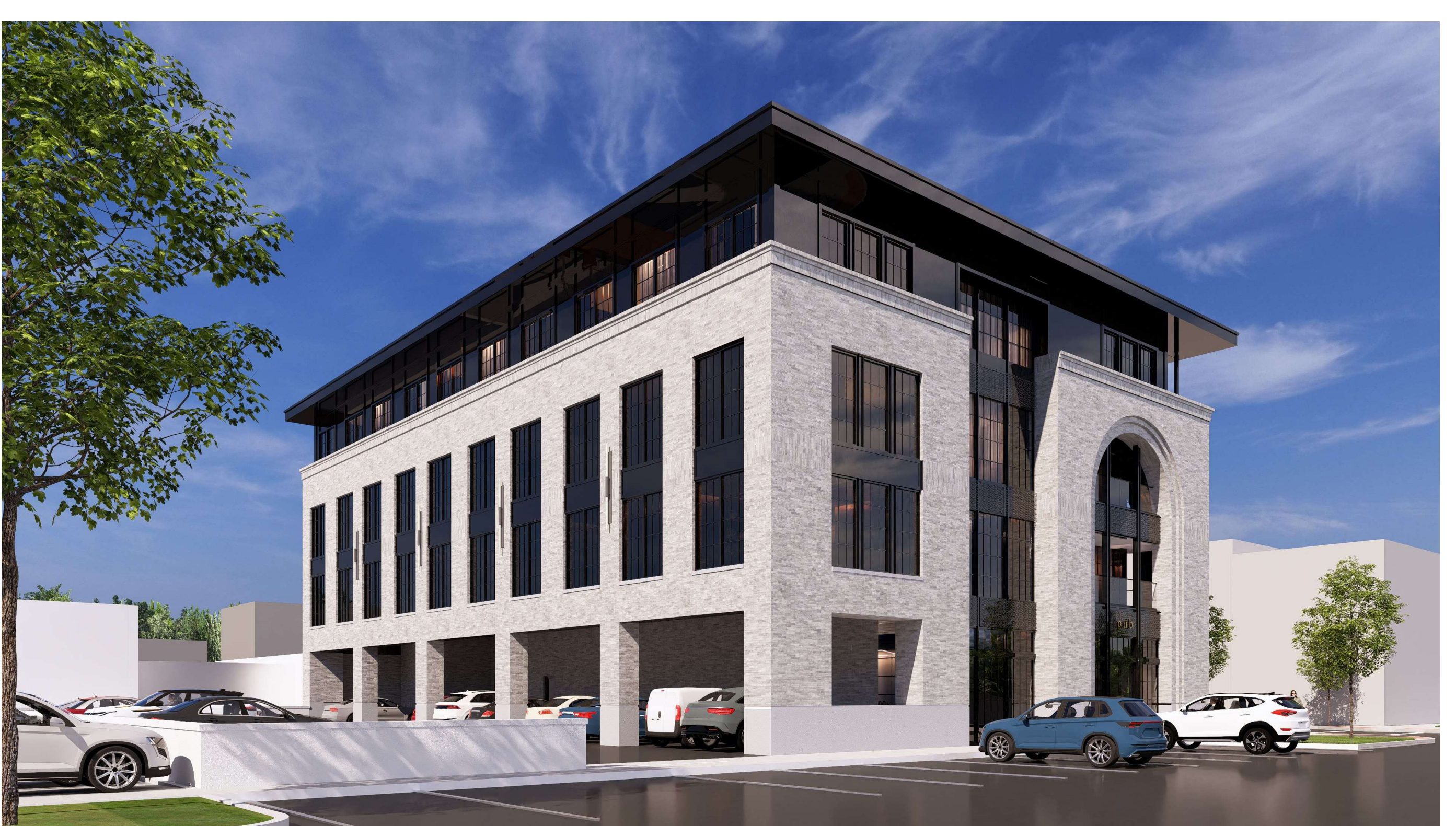
View of back facade
