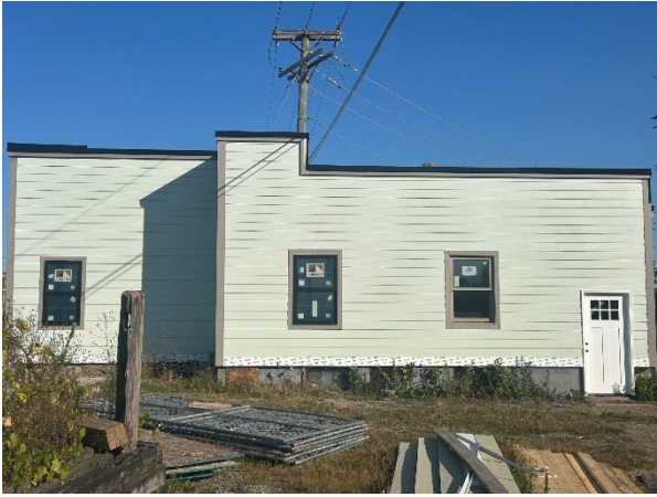
Roof Coping and Cap (finished 9.10.25)
