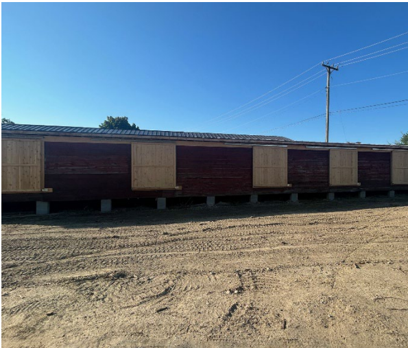
Structurally Rebuilt North Wall and Doors
