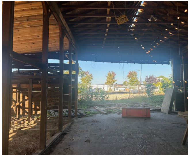
Footing repairs ongoing. The West and East Walls are intended to be rebuilt with original materials but to have glass panels for light and structure.
