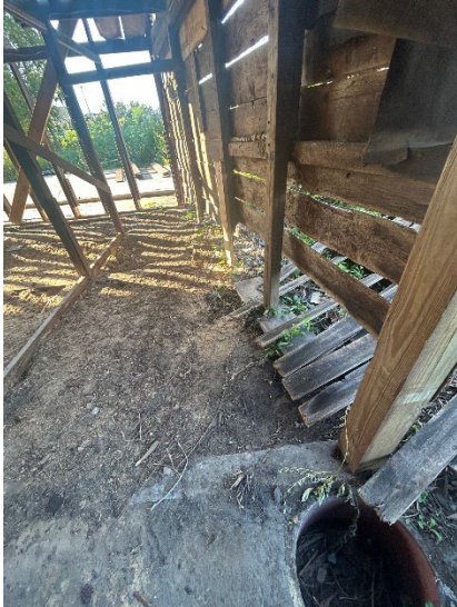
Footing repairs ongoing. The West and East Walls are intended to be rebuilt with original materials but to have glass panels for light and structure.
