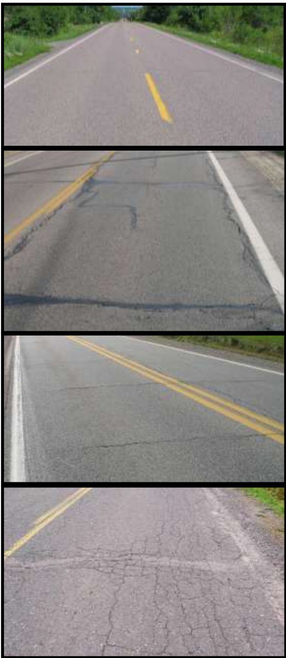
Figure 2: Top image – PASER 8 road that is considered “Good” by the TAMC exhibit only minor defects. Second image – PASER 5 road that is considered “Fair” by the TAMC. Exhibiting structural soundness but could benefit from CPM. Third image – PASER 6 road that is considered “Fair” by the TAMC. Bottom image – PASER 2 road that is considered “Poor” by the TAMC exhibiting significant structural distress.
