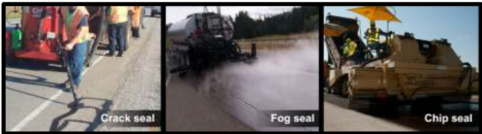
Figure 5: Examples of capital preventive maintenance treatments—(from left) crack seal, fog seal, chip seal
