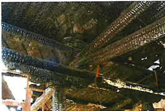
9. Close up view - charred wood beams
