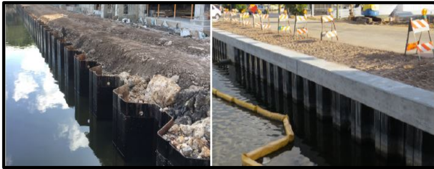
Steel Sheet Piles Bulkhead
