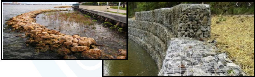
Combination Gabion Bulkhead & Living Shoreline
