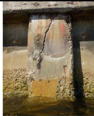
Photo E-55: Deterioration on soldier piles at the easement bulkhead.
