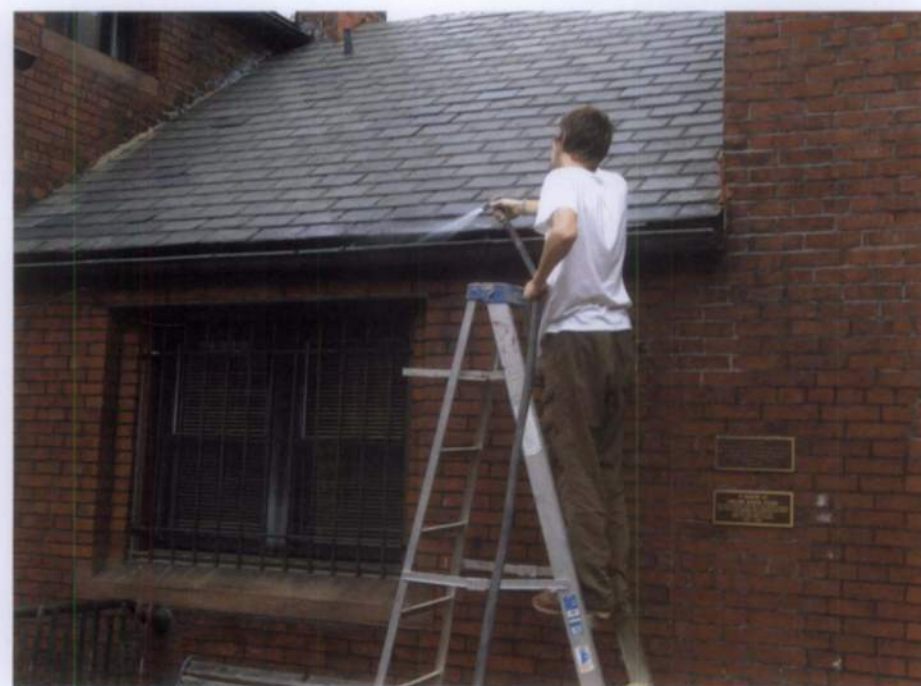
Figure 3. Keeping gutters clean of debris can be one of the most important cyclical maintenance activities. On this small one-story addition, a garden hose is being used to flush out the trough to ensure that the gutter and downspouts are unobstructed. Gutters on most small and medium size buildings can be reached with an extension ladder and a garden hose. Photo: Bryan Blumfeld.
