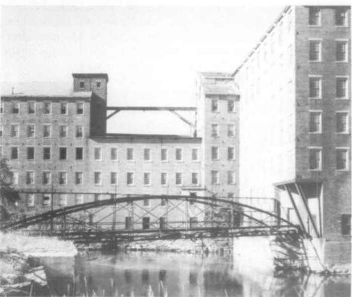
Figure 1. Windows are frequently important visual focal points, especially on simple facades such as this mill building. Replacement of the multi-pane windows here with larger panes could dramatically change the appearance of the building. The areas of missing windows convey the impression of such a change. Photo: John T. Lowe
