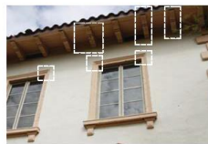
SOUTH ELEVATION: ROTTED RAFTER TAIL, CRACKED WINDOW EXTERIOR MOLDING
