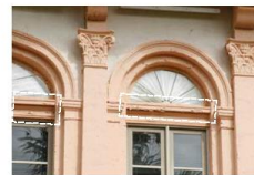
SOUTH ELEVATION: CHIPPED PAINT ON HEAD CASING. TYP. REFER TO A-21 AND A-22 WINDOWS FOR INSPECTION AND REPAIR GUIDELINES.
