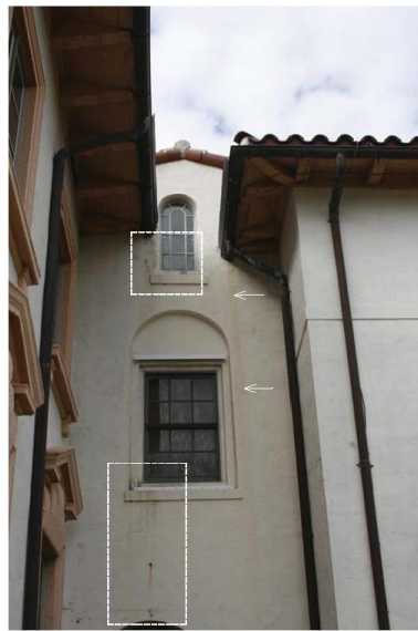
EAST ELEVATION: WATERMARKS AND LOCALIZED CLUSTERS OF MOLD. REFER TO A-20 EXTERIOR CLEANING AND A-24 STUCCO FOR STUCCO REPAIR AND COLOR APPLICATION.
