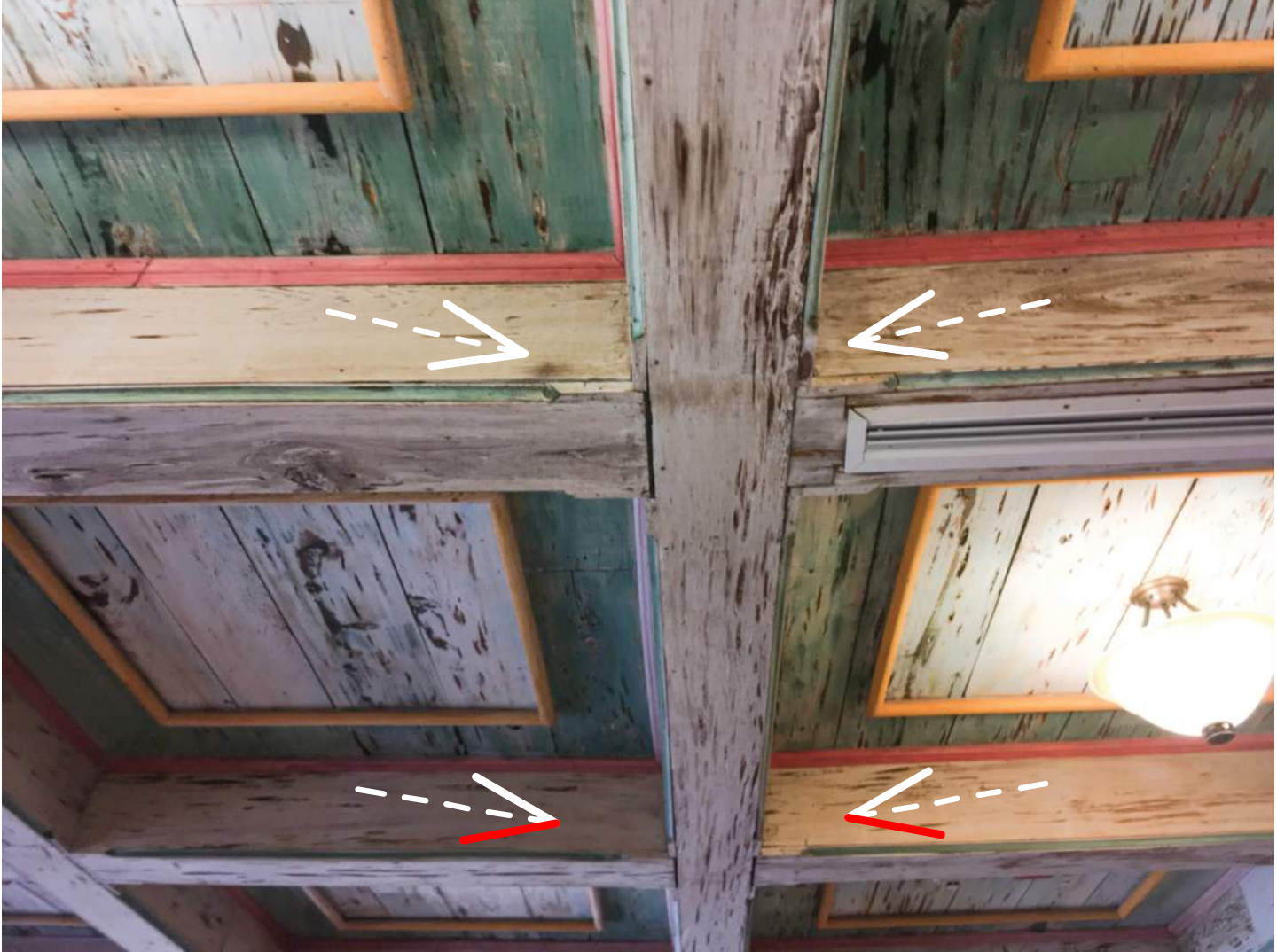
2 DETERIORATED COFFERED CEILING COMPONENTS; OVERALL SURFACE DECAY. REFFER TO SR-1, SR-2, SR-3, SR-4 STRUCTURAL REPORT.
