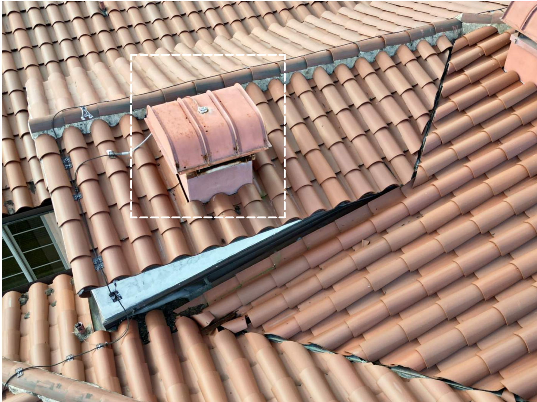
EXISTING ROOF EXHAUST VENT SHALL BE REMOVED
