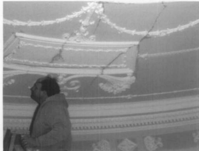
Fig. 6. Uninsulated plumbing pipes close to the exterior wall froze and cracked, wetting this ornamental plaster ceiling before the water supply line could be shut off. As a result, limited portions of the ceiling needed reattaching. Photo: author.
