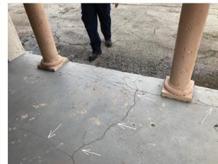
② NORTH ELEVATION: STRUCTURAL DAMAGE ON FLOOR SLAB. REFER TO S-4 CONCRETE REPAIRS' DETAILS AND PRODUCT SPECIFICATIONS.
