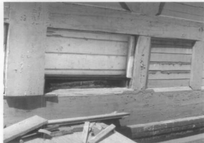
Fig. 8. Dampening moisture conditions can occur during construction. Peeling paint on this newly rehabilitated frame wall was attributed to wall insulation that had become wet during the project and was not discovered. Photo: NPS Files.
