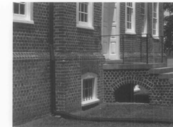
Fig. 17. In testing a theory for the cause of basement wetness, the owner used long black extender pipes to direct roof run-off away from the foundation. This test established that the owner did not need expensive waterproofing of the foundation, but a better drainage system. Photo: Baird M. Smith.
