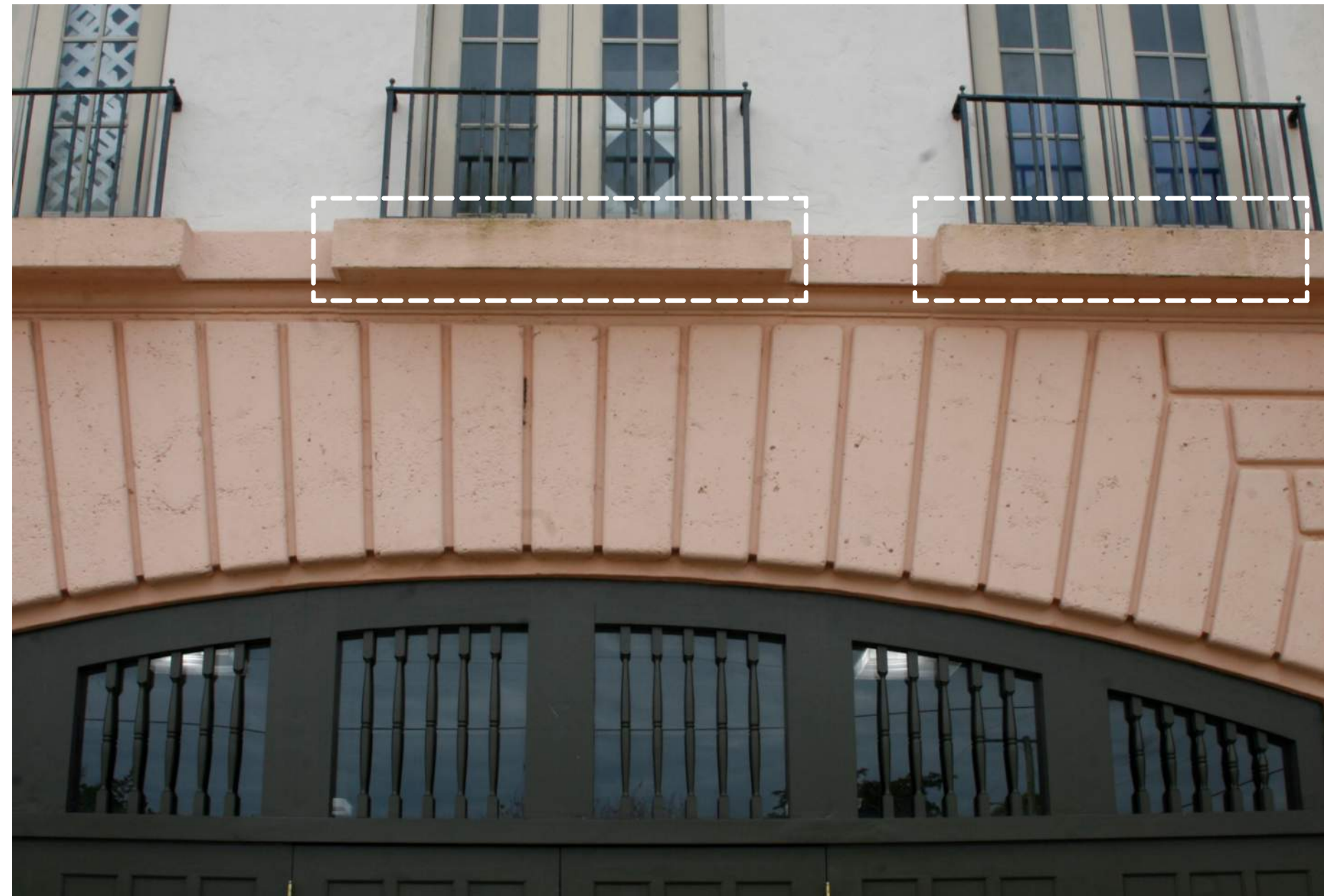
NORTH ELEVATION: FACADE DISCOLORATION. V.I.F.
