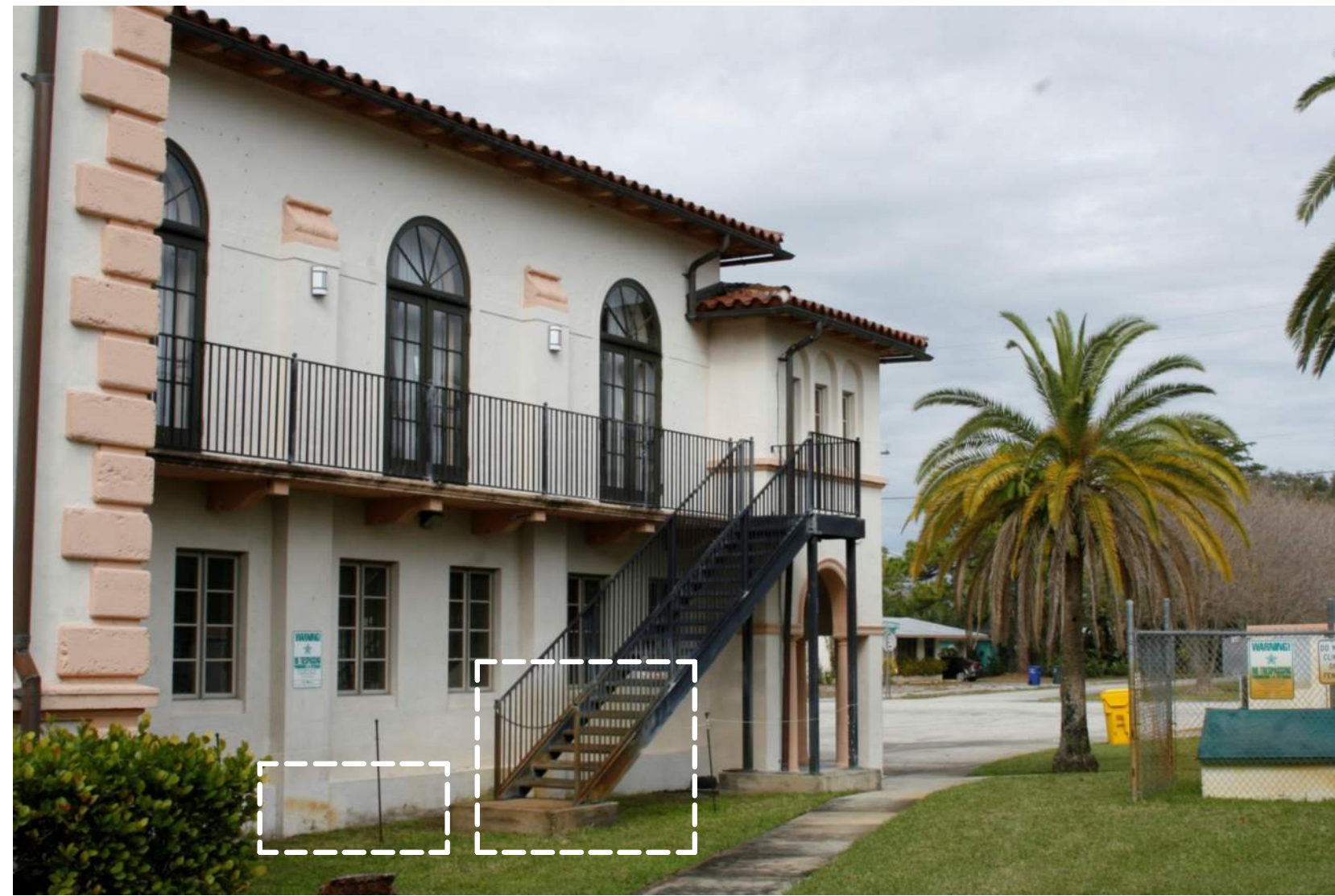
4 EAST ELEVATION: WATER DAMAGE ON FINISHED SURFACE. REFER A-23, A-24, A-25 STUCCO FOR STUCCO REPAIRS AND COLOR APPLICATION. REFER TO S-3 FOR STRUCTURAL REPAIRS ON BALCONY'S SLAB. PRESENCE OF RUST ON METAL STAIRS AND ASSOCIATED RAILING. REFER TO A-16c FOR EXTERIOR PAINT COATING SYSTEMS AND SURFACE PREPARATION.
