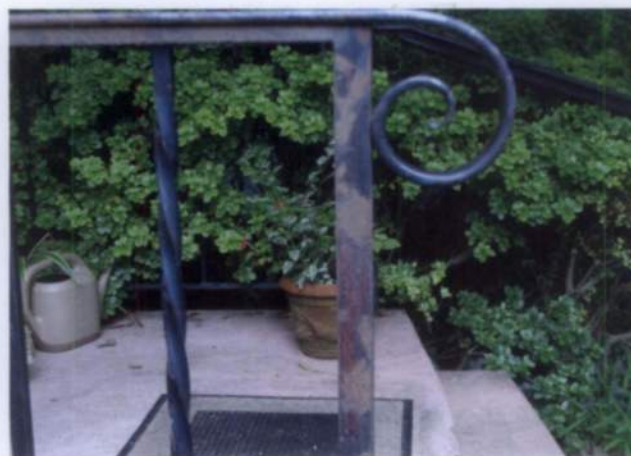
Figure 15. Metal projecting elements on a building, such as sign armatures and railings, are easily subject to rust and decay. Proper surface preparation to remove rust is essential. Special metal primers and topcoats should be used.
