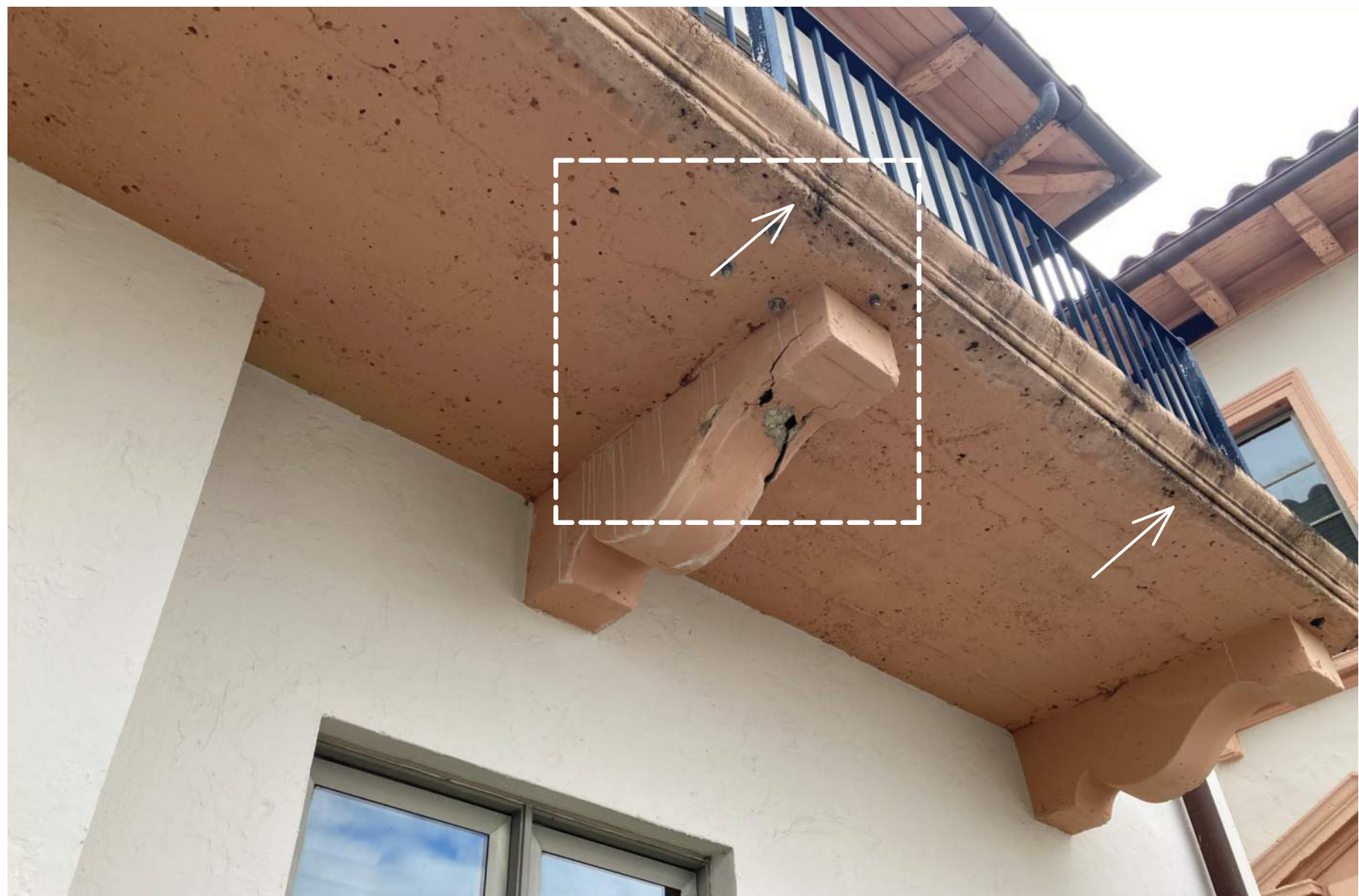
WEST ELEVATION: BUILD-UP OF MOLD ON SLAB. REFER TO A-20 EXTERIOR CLEANING. STRUCTURAL DAMAGED ON RAFTERTAIL. REFER TO S-4 CONCRETE REPAIRS' DETAILS AND PRODUCT SPECIFICATIONS.
