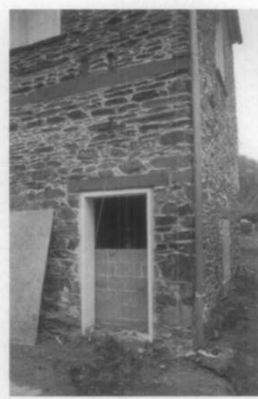
E. Mechanical systems on the lower level were placed on platforms above the flood line. Harper's Ferry Center, NPS.
