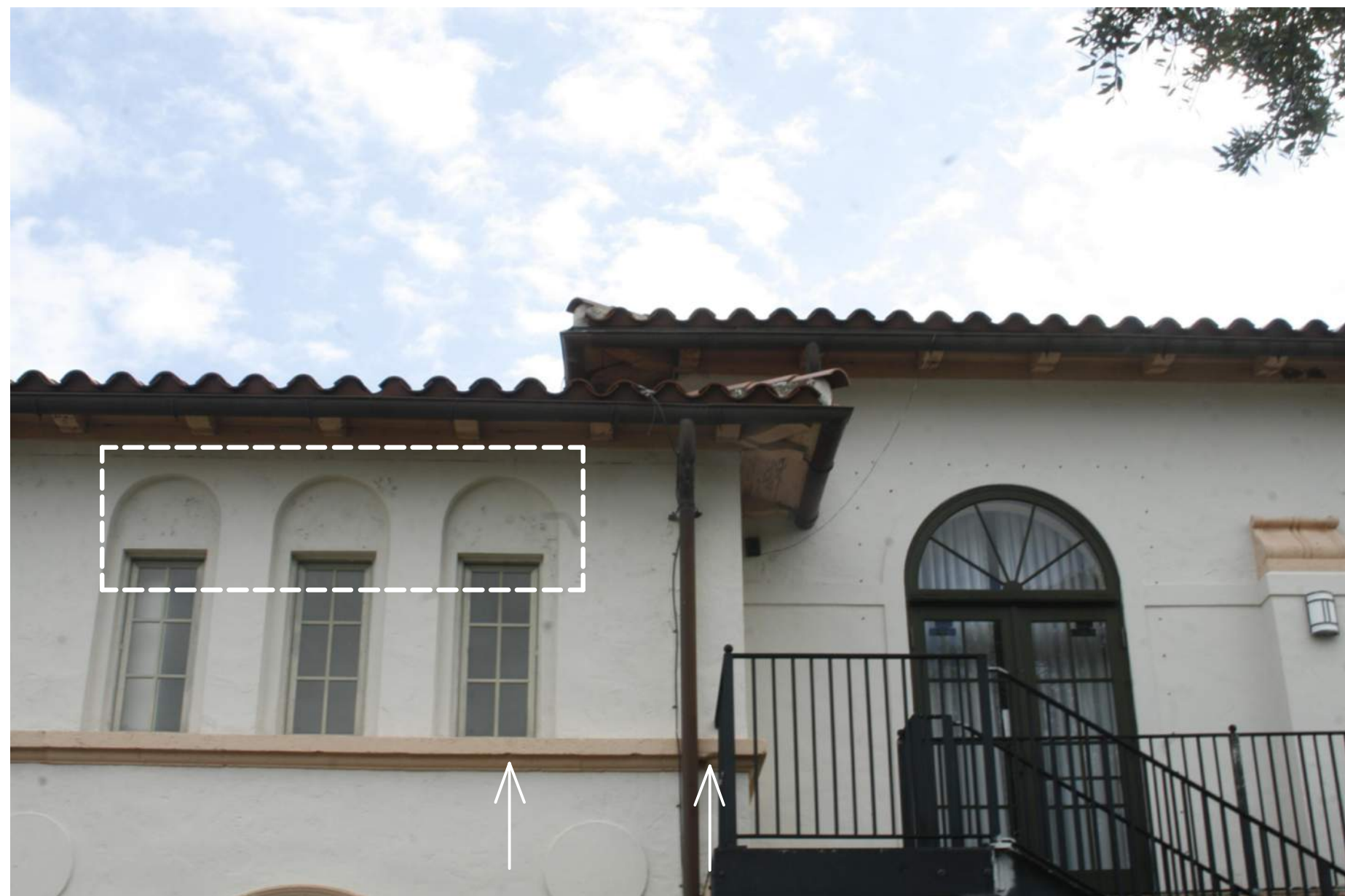
WEST ELEVATION: VERIFY CONDITION OF MOLDING. DETERIORATED STUCCO OR PAINT COAT. V.I.F. IF STUCCO, REFER TO A-23, A-24, A-25 STUCCO FOR STUCCO REPAIRS AND COLOR APPLICATION.
