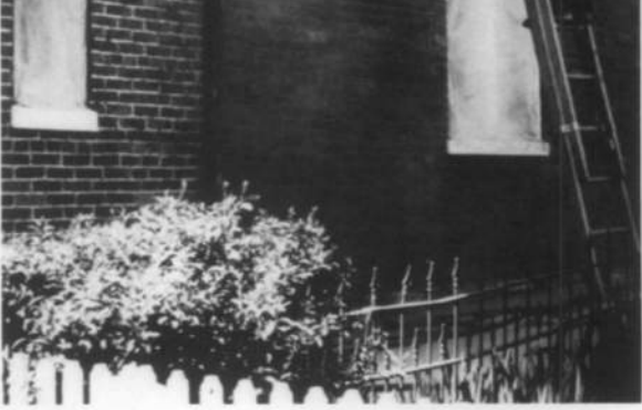
"Line Drop." Even though the operator of the sandblasting equipment is standing on a ladder to reach the higher sections of the wall, it is still almost impossible for him to control the pressure. The pressure of the sand hitting the lower portion of the wall will still be greater than that above, because of the "line drop" in the distance from the pressure source to the nozzle. (Hugh Miller)
