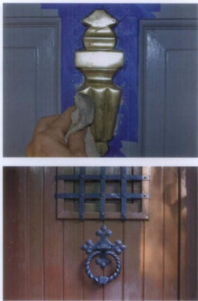
Figure 1. Maintenance involves selecting the proper treatment and protecting adjacent surfaces. Using painter's tape to mask around a brass doorknocker protects the painted door surface from damage when polishing with chemical compounds. On the other hand, hardware with a patinated finish was not intended to be polished and should simply be cleaned with a damp cloth.
