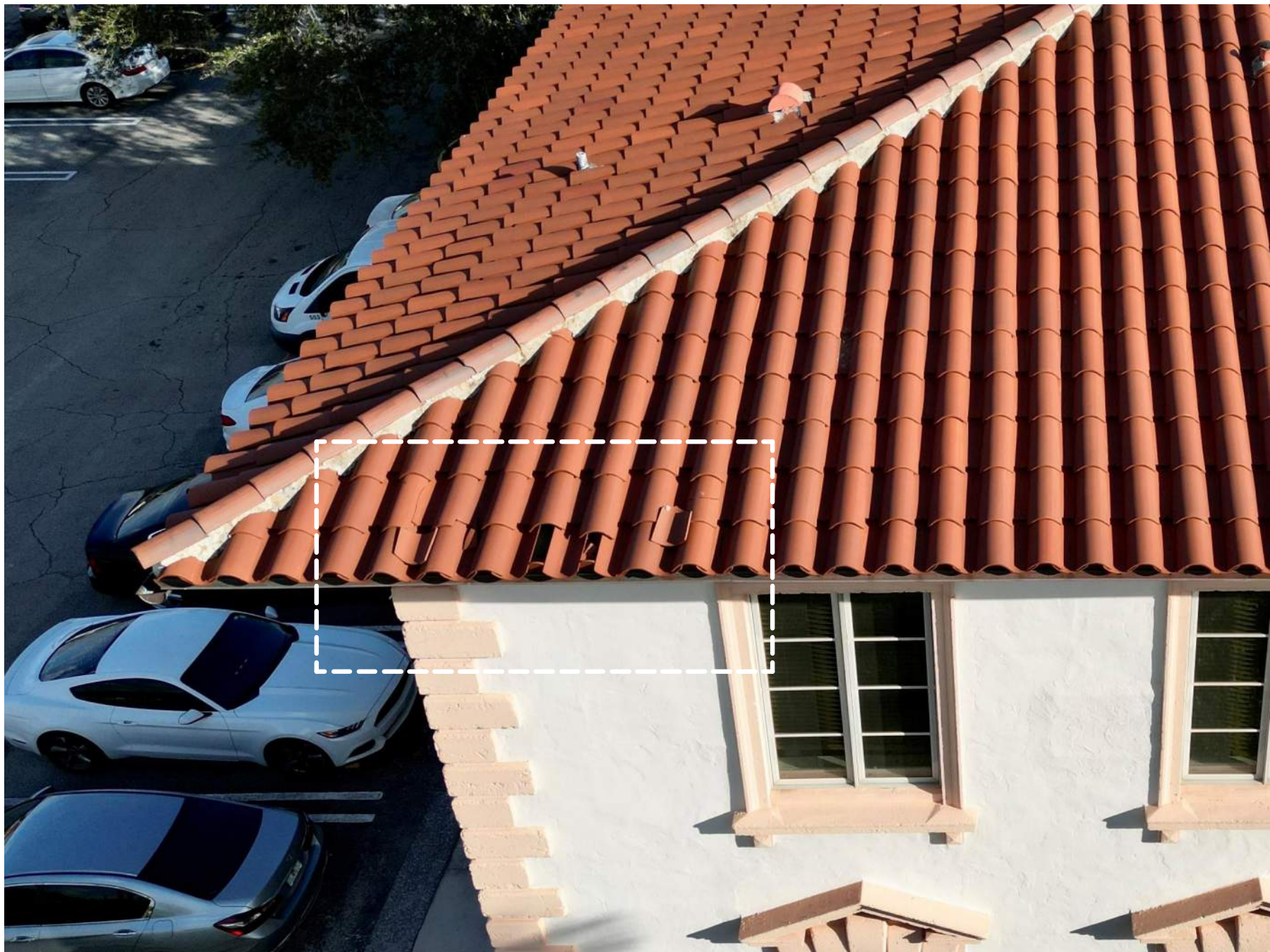
PARTIAL DAMAGE (EXPOSED ROOF)
