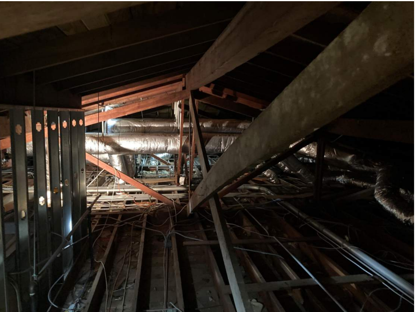
WOOD ROOF FRAMING STRUCTURE W/ WOOD ROOF TRUSSES
