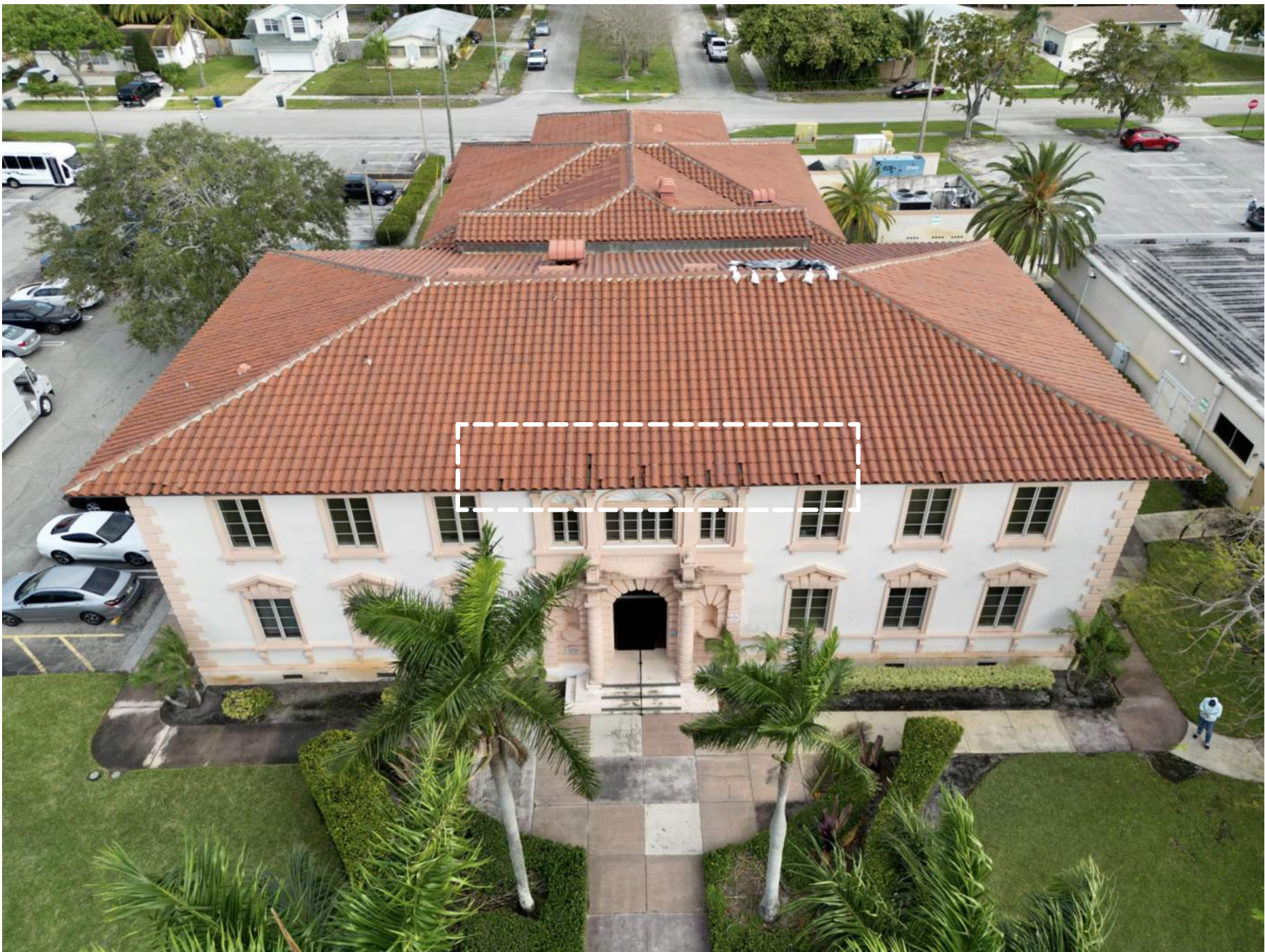
MAIN ENTRANCE: SOUTH AERIAL VIEW ROOF CONDITION, MISSING ROOF TILES.
