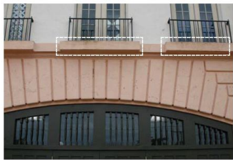
NORTH ELEVATION: FACADE DISCOLORATION. V.I.F.
