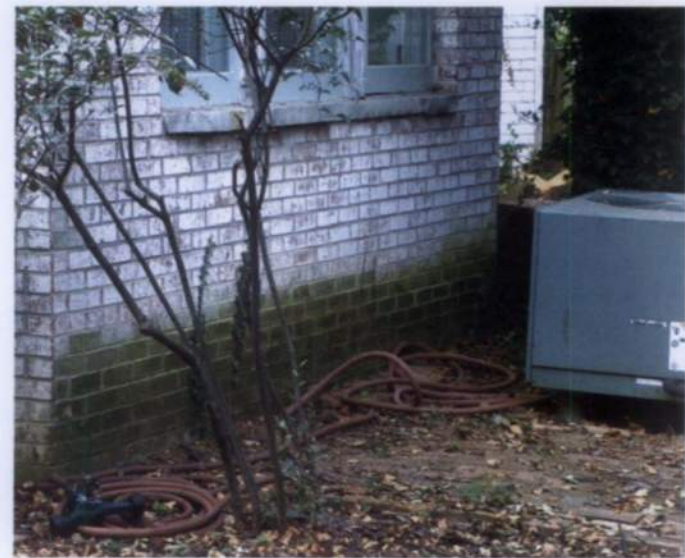
Figure 17. Extending downsouts at their base is one of the basic steps to reduce dampness in basements, crawl spaces and around foundations. Extensions should be buried. If possible, for aesthetics, ease of lawn care, and to avoid creating a tripping hazard.
