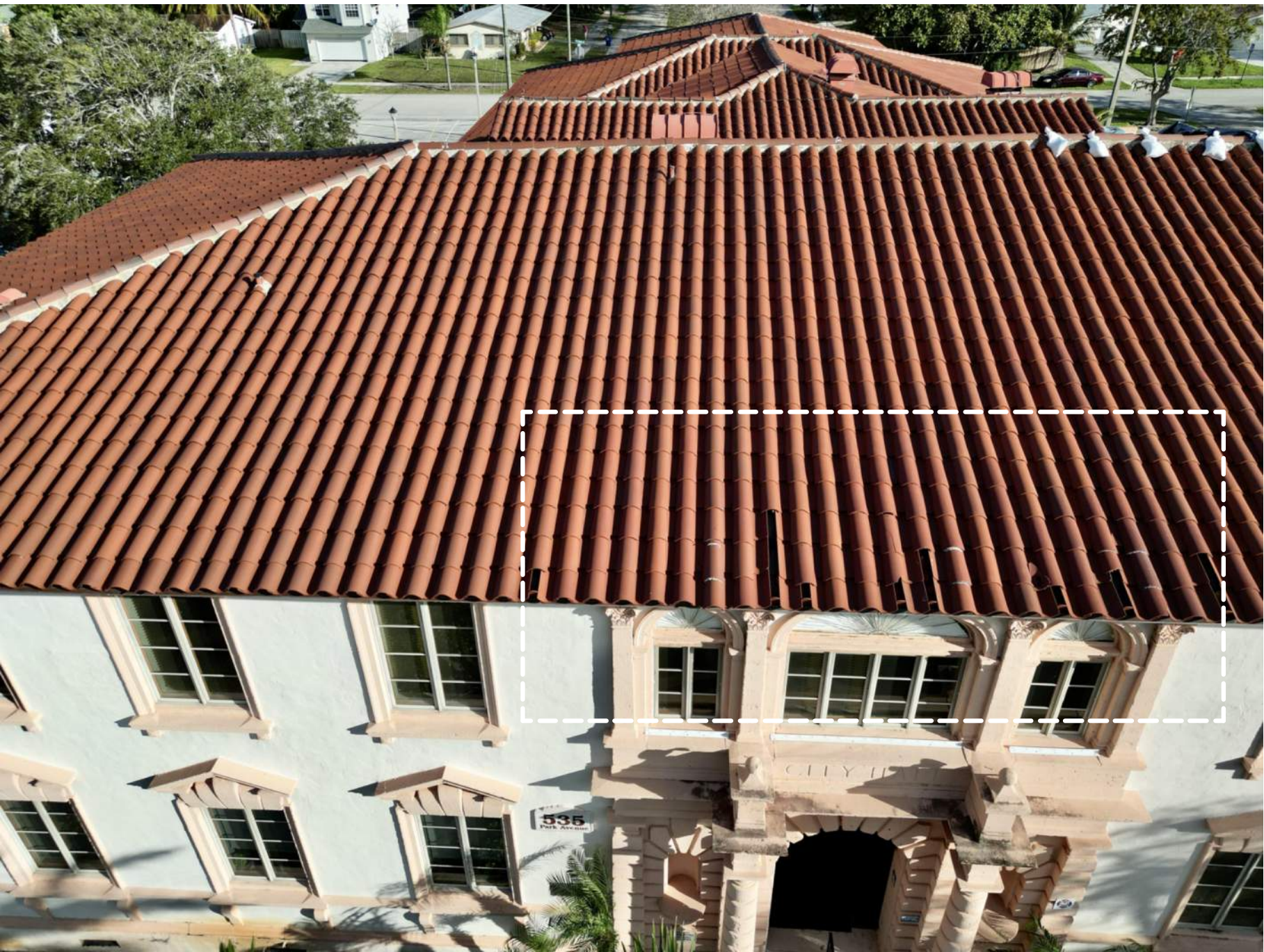
SOUTH AERIAL ROOF VIEW / MISSING AND CHIPPED ROOF TILES, REMOVE ALL VENTS AS REQUIRED.
