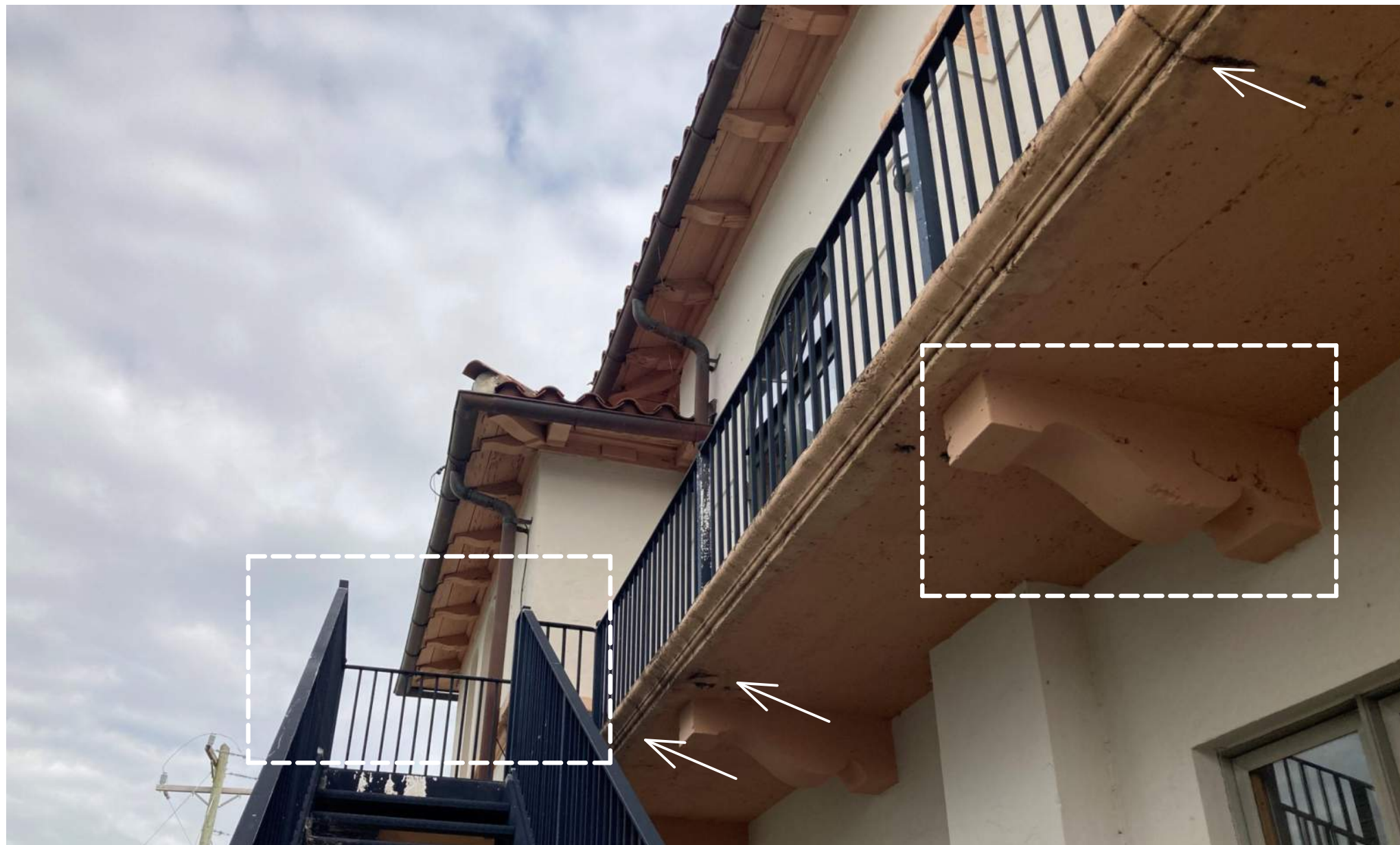
WEST ELEVATION: STRUCTURAL DAMAGED ON RAFTERTAIL AND BALCONY SLAB. REFER TO S-4 CONCRETE REPAIRS' DETAILS AND PRODUCT SPECIFICATIONS. V.I.F. REFER TO S-2 IF DAMAGE ON BALCONY SLAB IS PRESENT. PRESENCE OF RUST ON METAL STAIRS AND ASSOCIATED RAILING. REFER TO A-16c FOR EXTERIOR PAINT COATING SYSTEMS AND SURFACE PREPARATION.
