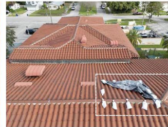
LEAKAGE ON EXISTING ROOF, WATER INTRUSION
