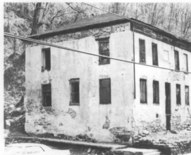
Fig. 7. Patches of stucco have fallen off this derelict 19th century structure exposing the rough-cut local stone substrate. The missing wood entablature on the side and the rough wood lintel now exposed above a second-floor window, offer clues that the building was stuccoed originally. Photo: National Park Service Files.
