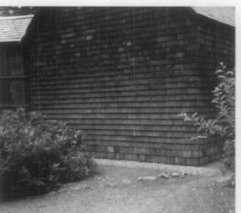
C. The new ground gutter gravel base helps drainage around the concrete foundation (see B above) which is not visible behind the replaced wooden wall shingles. Photo: WPTC, NPS.
