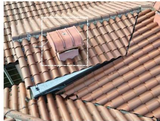
EXISTING ROOF EXHAUST VENT SHALL BE REMOVED
