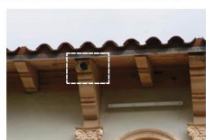
SOUTH ELEVATION: FOREIGN OBJECT EMBEDDED ON RAFTER TAIL. V.I.F. REMOVE AND REPAIR RAFTER TAIL.
