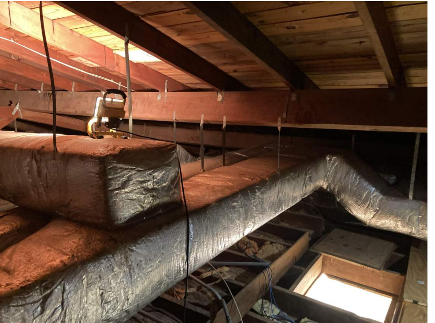
DUCT SYSTEM UNDER ROOF BEAMS
