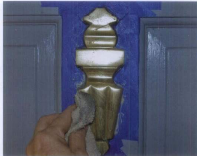
Figure 1. Maintenance involves selecting the proper treatment and protecting adjacent surfaces. Using painter's tape to mask around a brass doorknocker protects the painted door surface from damage when polishing with chemical compounds. On the other hand, hardware with a patinated finish was not intended to be polished and should simply be cleaned with a damp cloth.
