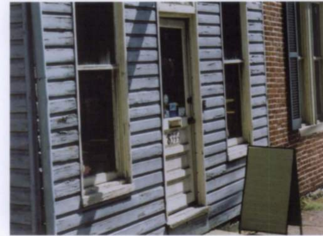
Figure 8. The paint on the siding of this south-facing wall needs to be scraped, sanded, primed and repainted. Postponing such work will lead to further paint failure, greater water penetration, and possibly even result in the need to replace some siding. Photo: Charles Fisher.
