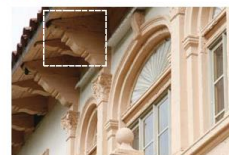
SOUTH ELEVATION: DETERIORATION OF PAINT COAT ON RAFTER TAILS. REPAIR AS NECESSARY.
