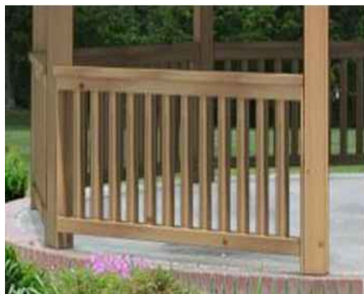
Square Railing 2"x2" Pickets 4" On center 32" Height
