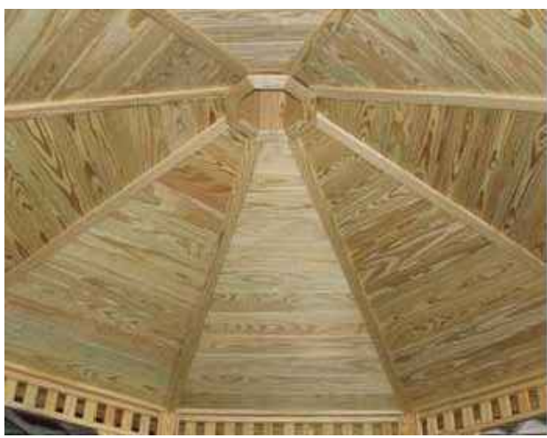
Finished Ceiling 1"x6" T&G PT Pine Boards Boards Covered With 1"x3" Trim Trim Boards Over All Seams And Around Any Openings #1 Kiln Dried PT Pine With SS Screws and Fasteners Throughout
