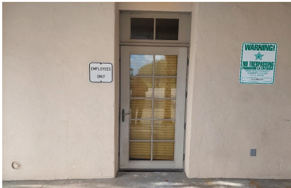
Single Door Entry at rear of Town Hall into Public Information Office Door to be replaced with similar door, Impact Rated with period correct aesthetics Reuse existing hardware
