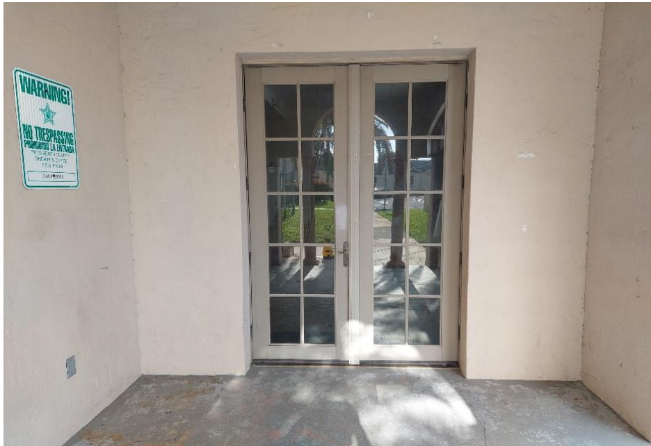
Double Door Entry at rear of Town Hall Commission Chambers Doors to be replaced with similar door, Impact Rated with period correct aesthetics Reuse existing hardware
