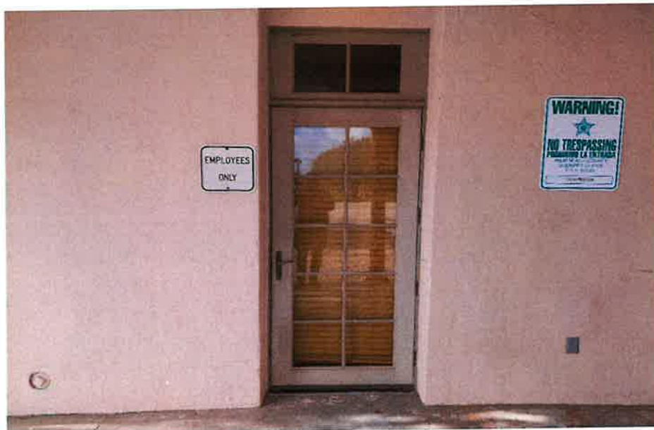
Single Door Entry at rear of Town Hall into Public Information Office Door to be replaced with similar door, Impact Rated with period correct aesthetics Reuse existing hardware
