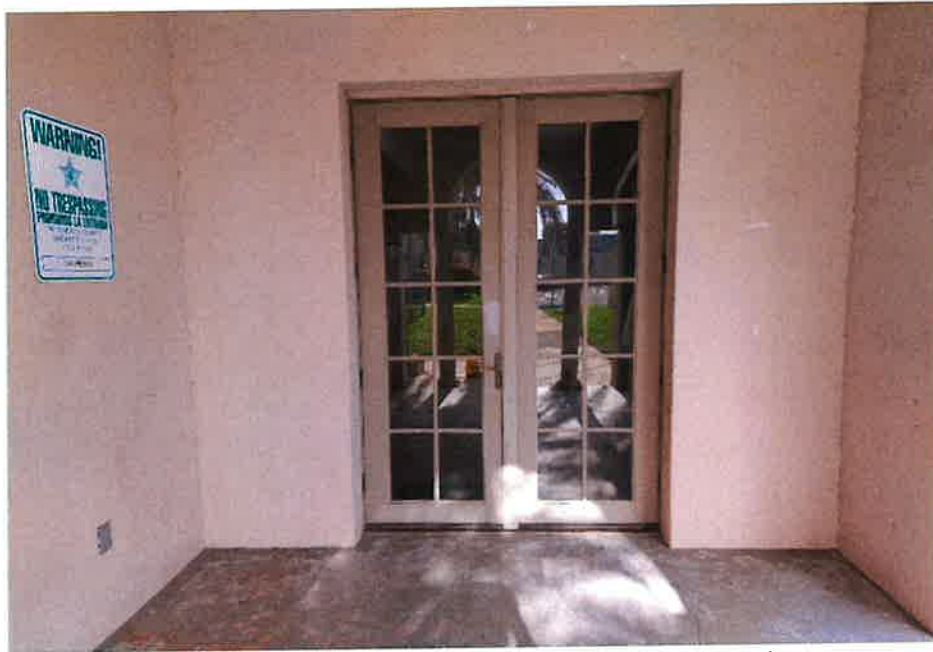
Double Door Entry at rear of Town Hall Commission Chambers Doors to be replaced with similar door, Impact Rated with period correct aesthetics Reuse existing hardware
