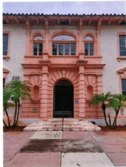
The sections of radius arched windows (above the casement windows) are not impact rated. Building exterior hardening plan is to change these openings to achieve an impact rating.
