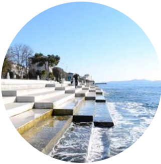
Stepped Concrete Seawall
