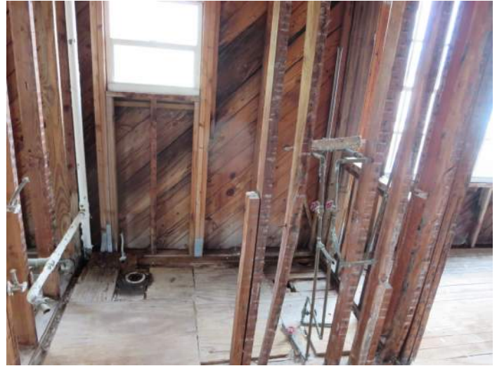
Discontinuous floor deck sheathing PHOTO NO. IMG_8002
