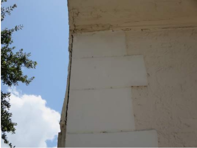
Finish separation PHOTO NO. IMG_7919
