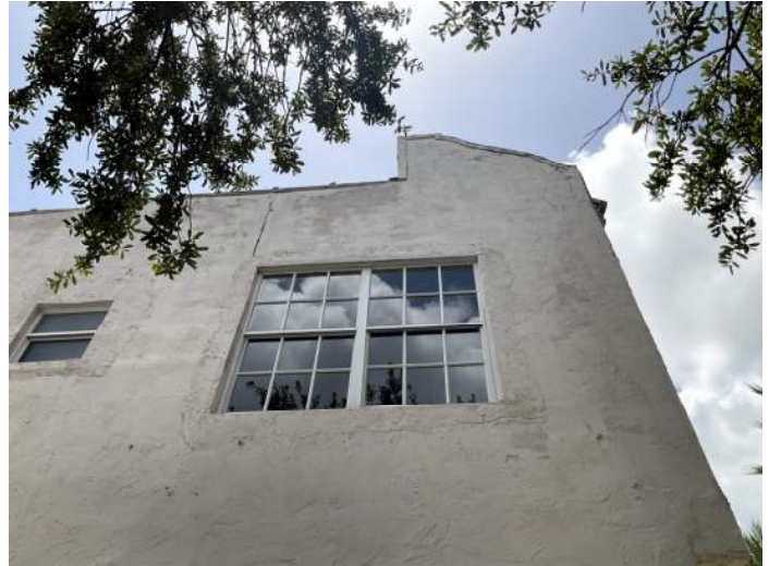
Stucco repair transition around window PHOTO NO. 20230710_175305873
