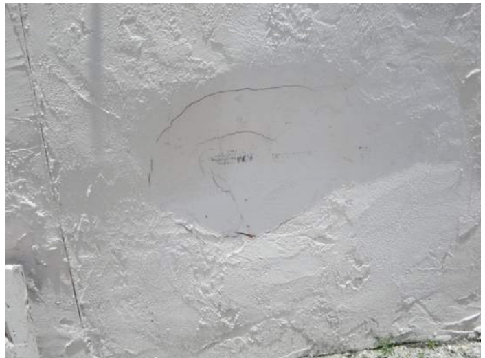
Stucco finish indentation PHOTO NO. IMG_7931
