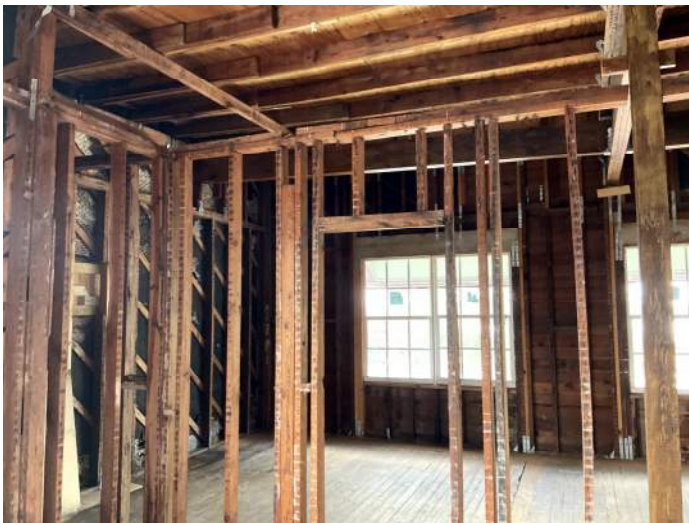
2 nd Floor interior wall framing PHOTO NO. 20230710_182257563
