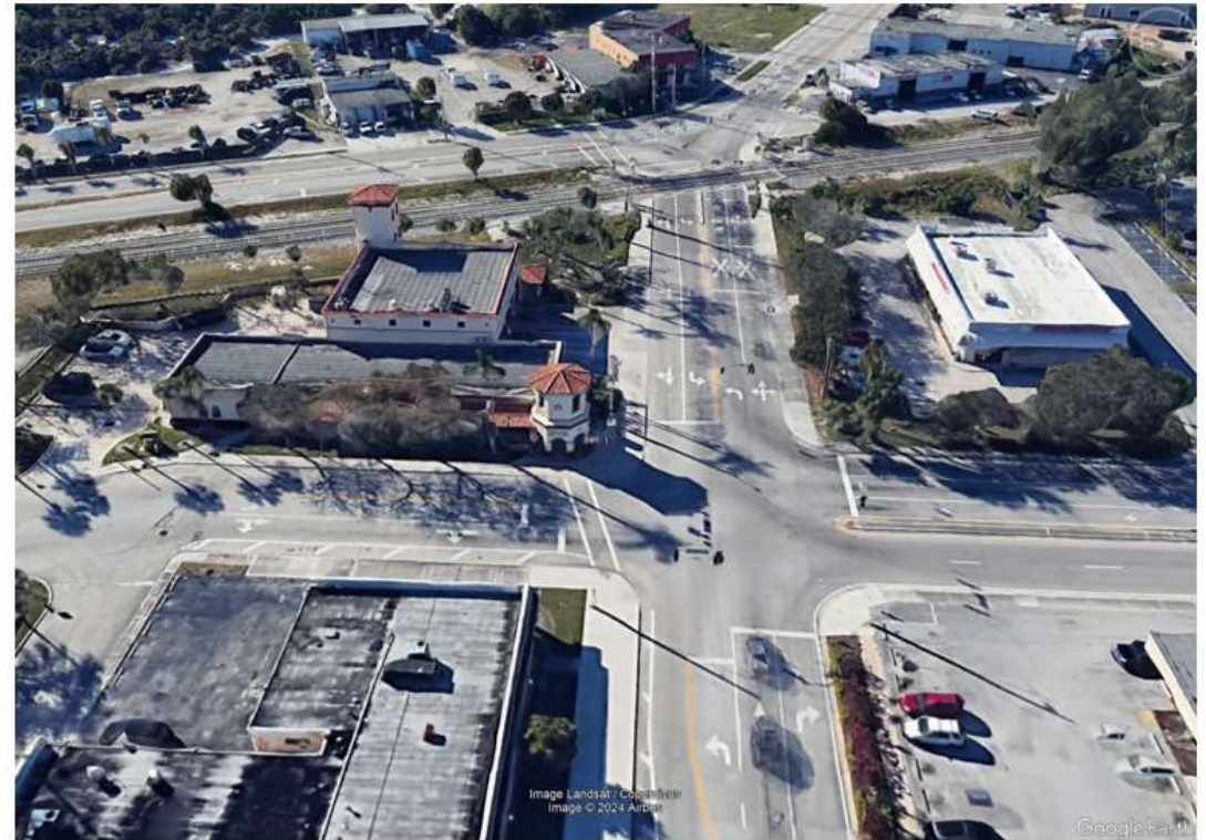
TRAFFIC: INTERSECTION AT PARK AVE. AND 10 TH ST.- COMPLICATED BY PROXIMITY OF RAILROAD TRACKS
