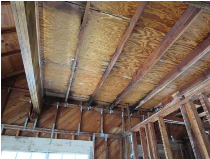
Roof framing and water stains at roof deck sheathing PHOTO NO. IMG_7999
