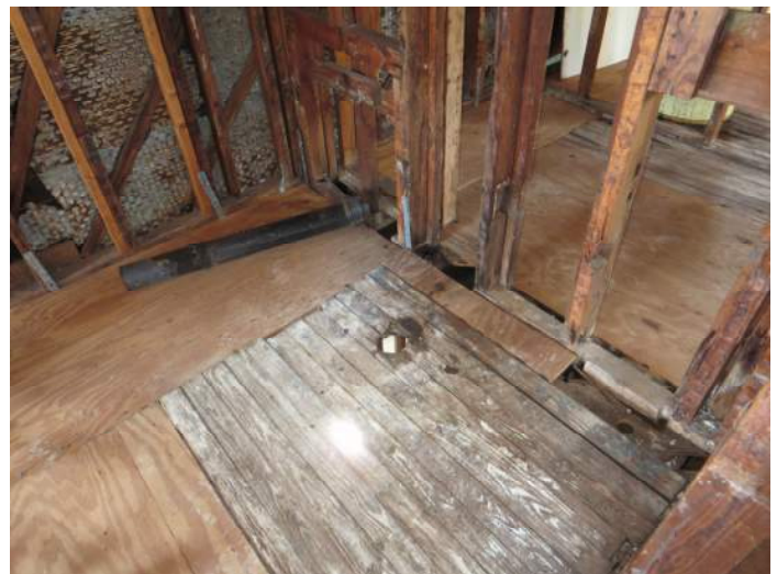
Discontinuous floor deck sheathing PHOTO NO. IMG_8011
