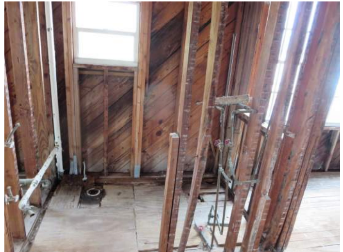
Discontinuous floor deck sheathing PHOTO NO. IMG_8002
