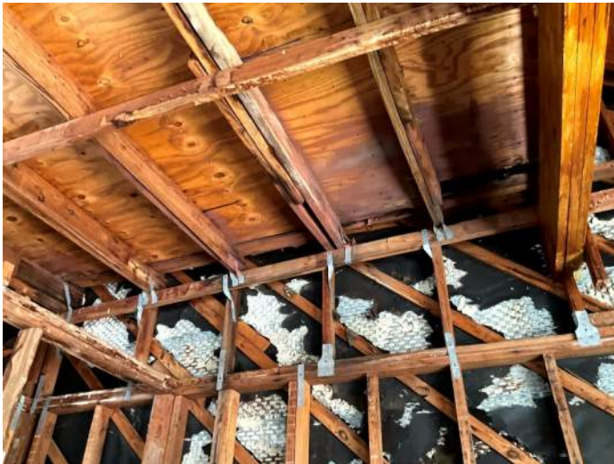
Spliced roof joist framing at bearing ends PHOTO NO. 20230710_182352450
