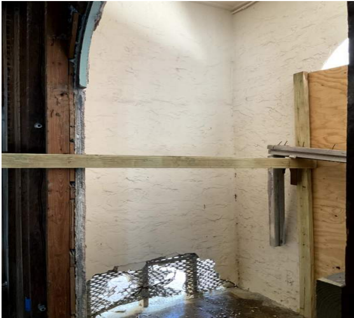
Spalled stucco finish PHOTO NO. 20230710_181632154
