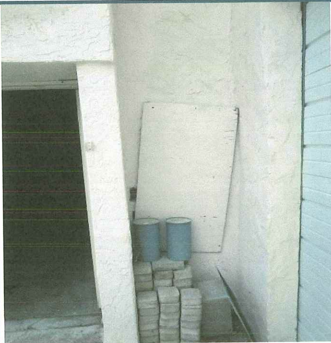
Unfastened board at wall opening PHOTO NO. IMG_7946
