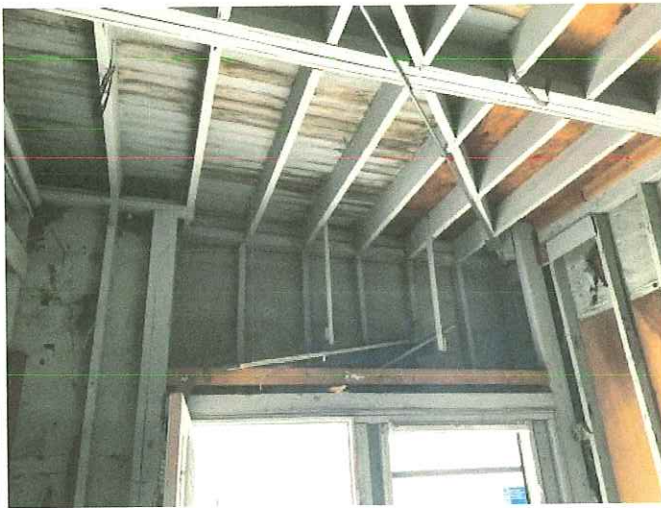
Rear expansion floor framing from underside PHOTO NO. 20230710_175601186
