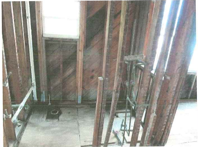
Discontinuous floor deck sheathing PHOTO NO. IMG_8002
