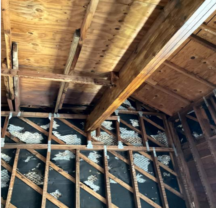
Unconventional top of wall framing PHOTO NO. 20230710_182333863
