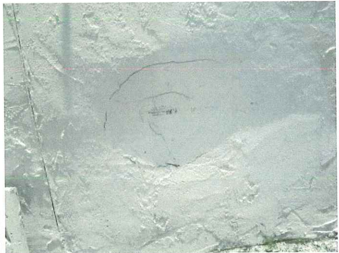
Stucco finish indentation PHOTO NO. IMG_7931
