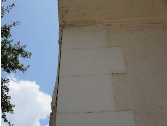
Finish separation PHOTO NO. IMG_7919
