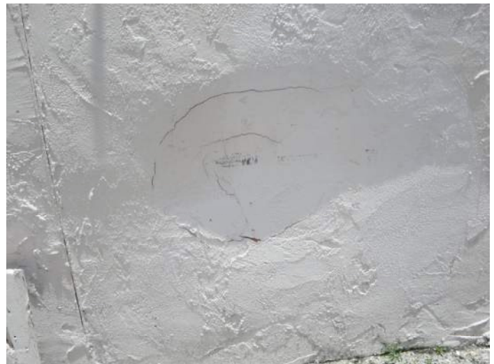
Stucco finish indentation PHOTO NO. IMG_7931
