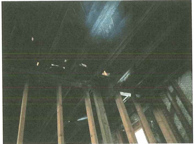
Underside of 2 nd floor framing, discontinued top plate PHOTO NO. 20230710_180448544
