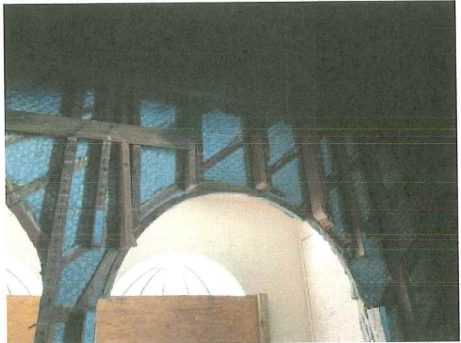
Missing header over arched openings PHOTO NO. 20230710_181658453
