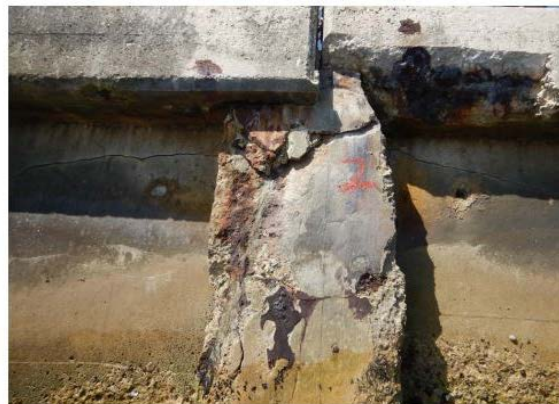
Photo E-56: Deterioration on soldier piles at the easement bulkhead.
