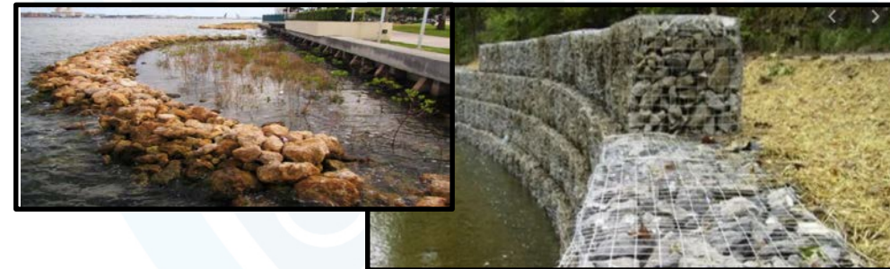
Combination Gabion Bulkhead & Living Shoreline
