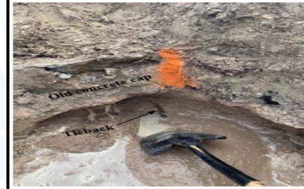
Photo A-70: An old bulkhead was revealed behind the existing bulkhead. A tieback was revealed at station 1+34.
