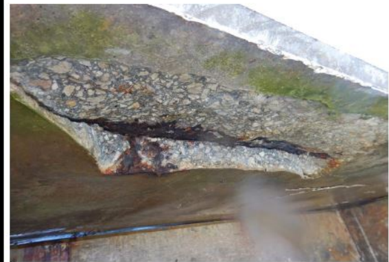
Photo A-40: Delamination at the bottom of the concrete slab between bent 14 and bent 14-a.
