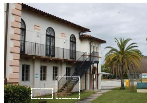
④ EAST ELEVATION: WATER DAMAGE ON FINISHED SURFACE. REFER: A-23, A-24, A-25 STUCCO FOR STUCCO REPAIRS AND COLOR APPLICATION. REFER TO S-3 FOR STRUCTURAL REPAIRS ON BALCONY'S SLAB. PRESENCE OF RUST ON METAL STAIRS AND ASSOCIATED RAILING. REFER TO A-16c FOR EXTERIOR PAINT COATING SYSTEMS AND SURFACE PREPARATION.
