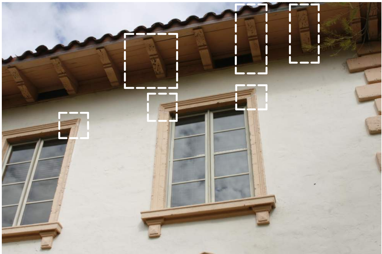
SOUTH ELEVATION: ROTTED RAFTER TAIL. CRACKED WINDOW EXTERIOR MOLDING
