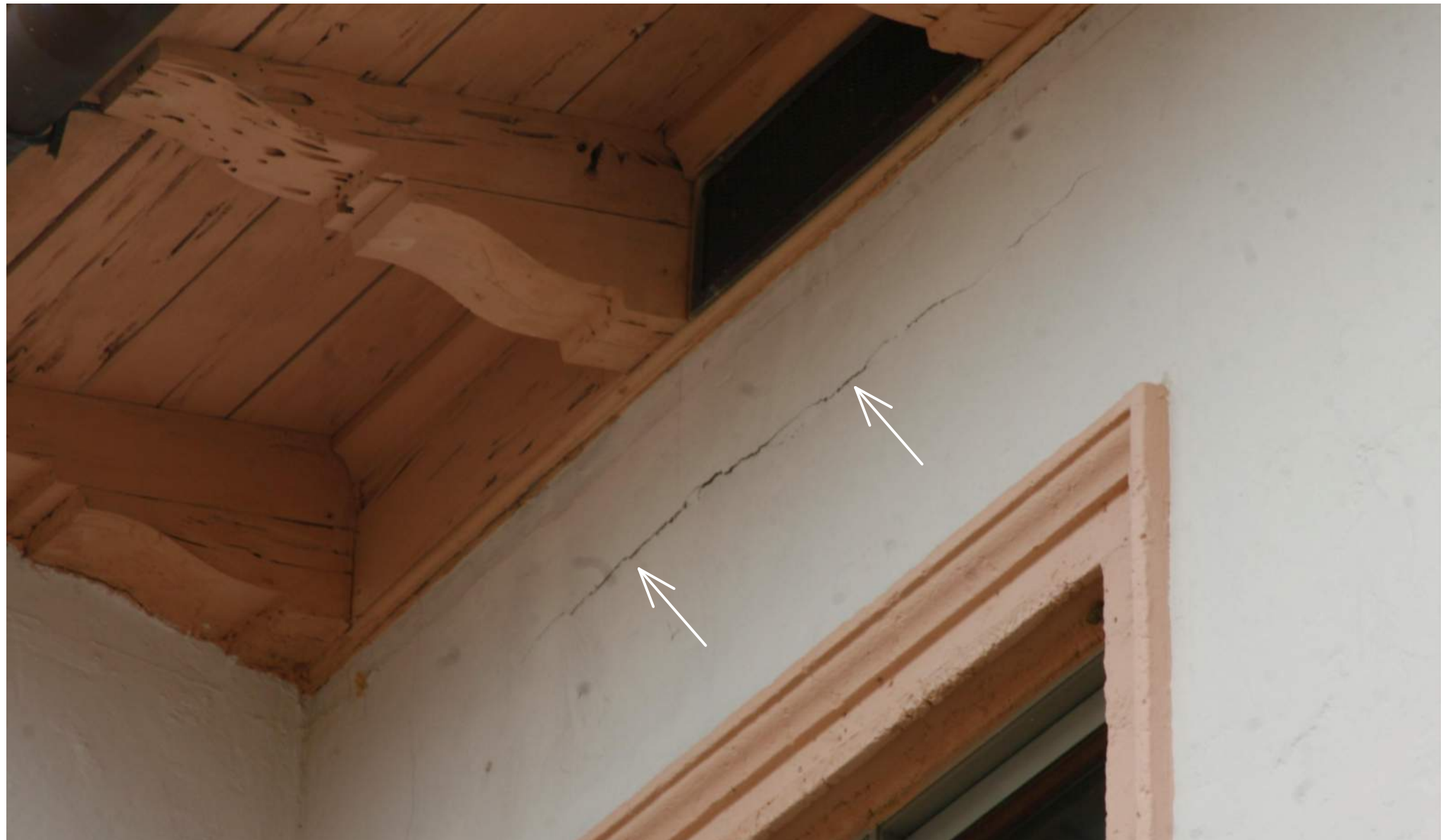
SOTH ELEVATION: DAMAGE ON FINISH COAT. ASSESS THE EXTENT OF DAMAGED AND INTEGRITY OF THE AREA IN THE FIELD. TYP. REFER TO SHEETS A-23, A-24 AND A-25 STUCCO.
