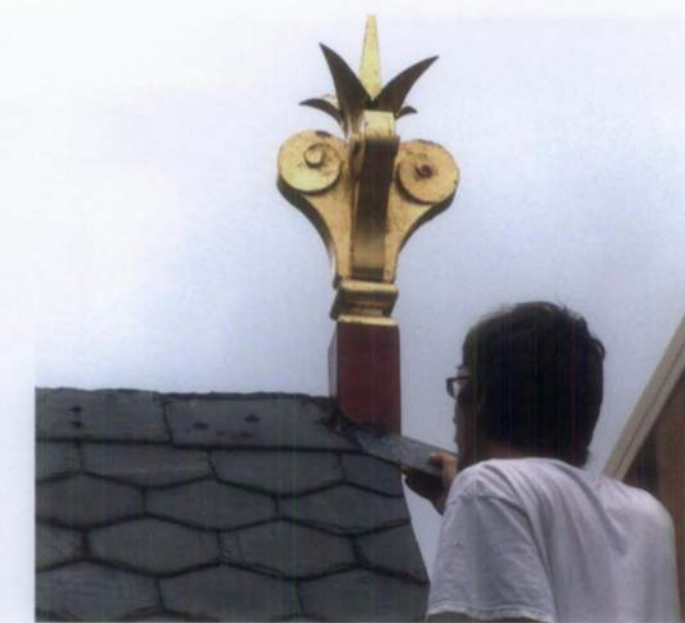
Figure 5. The use of a sealant to close an exposed joint is not always an effective long-term solution. Where this decorative wood element connects to the slate roof, the sealant has failed within a short time and a proper metal flashing collar is being fitted instead. Photo: Bryan Blumfeld.
