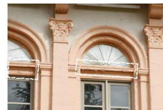
SOUTH ELEVATION: CHIPPED PAINT ON HEAD CASING. TYP. REFER TO A-21 AND A-22 WINDOWS FOR INSPECTION AND REPAIR GUIDELINES.
