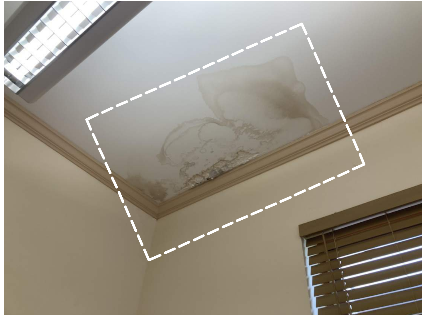
4 WATER DAMAGE ON CEILING. REFER TO A-26, A-27, A-28, A-29, A-30, A-31 MOISTURE CONTROL.
