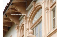
SOUTH ELEVATION: DETERIORATION OF PAINT COAT ON RAFTER TAILS. REPAIR AS NECESSARY.
