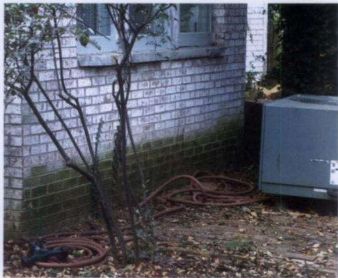
Figure 17. Extending downspouts at their base is one of the basic steps to reduce dampness in basements, crawl spaces and around foundations. Extensions should be buried, if possible, for aesthetics, ease of lawn care, and to avoid creating a tripping hazard.
