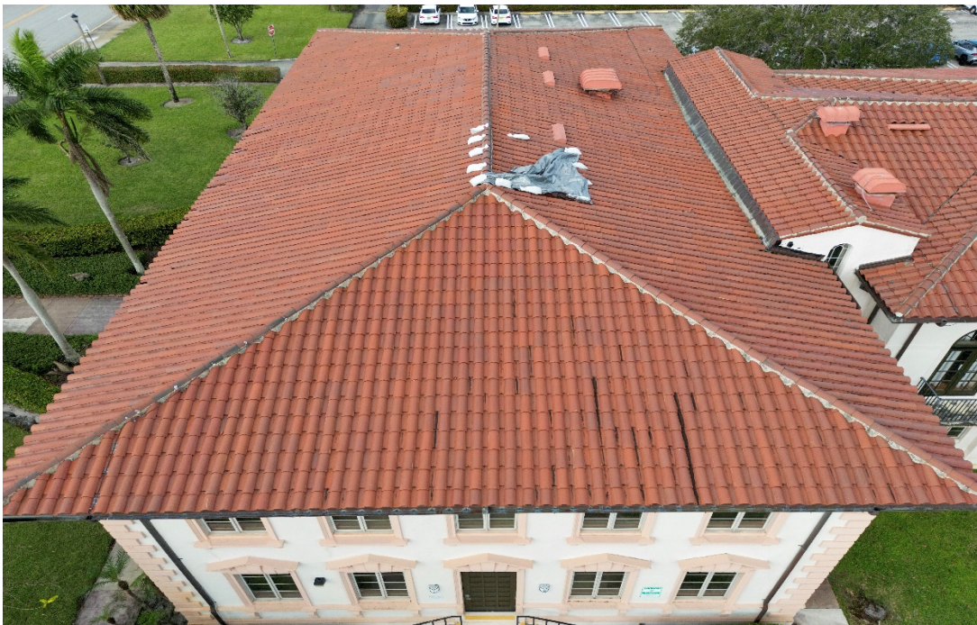
East side view of Town Hall Building Roof tile damage along roof ridge
