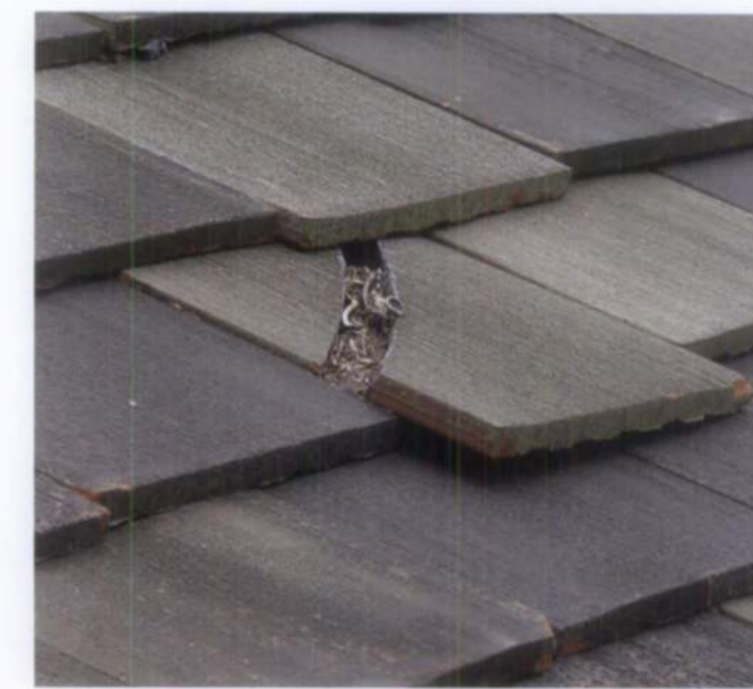
Figure 4. Damage to roofs often requires immediate attention. As a temporary measure, this damaged roof tile could be replaced with a brown aluminum sheet wedged between the existing tiles. Photo: Chad Randt.
