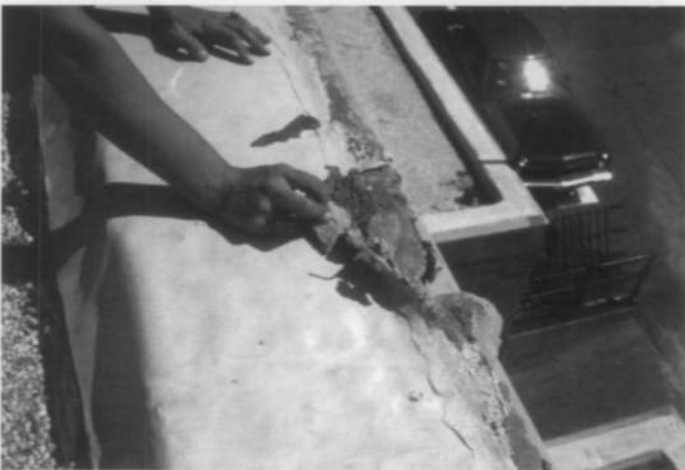
Fig. 1. Moisture problems, if not properly corrected, will increase damage to historic buildings. This waterproofing coating trapped moisture from the leaking roof, causing portions of the masonry parapet to fail. Photo: NPS Files.
