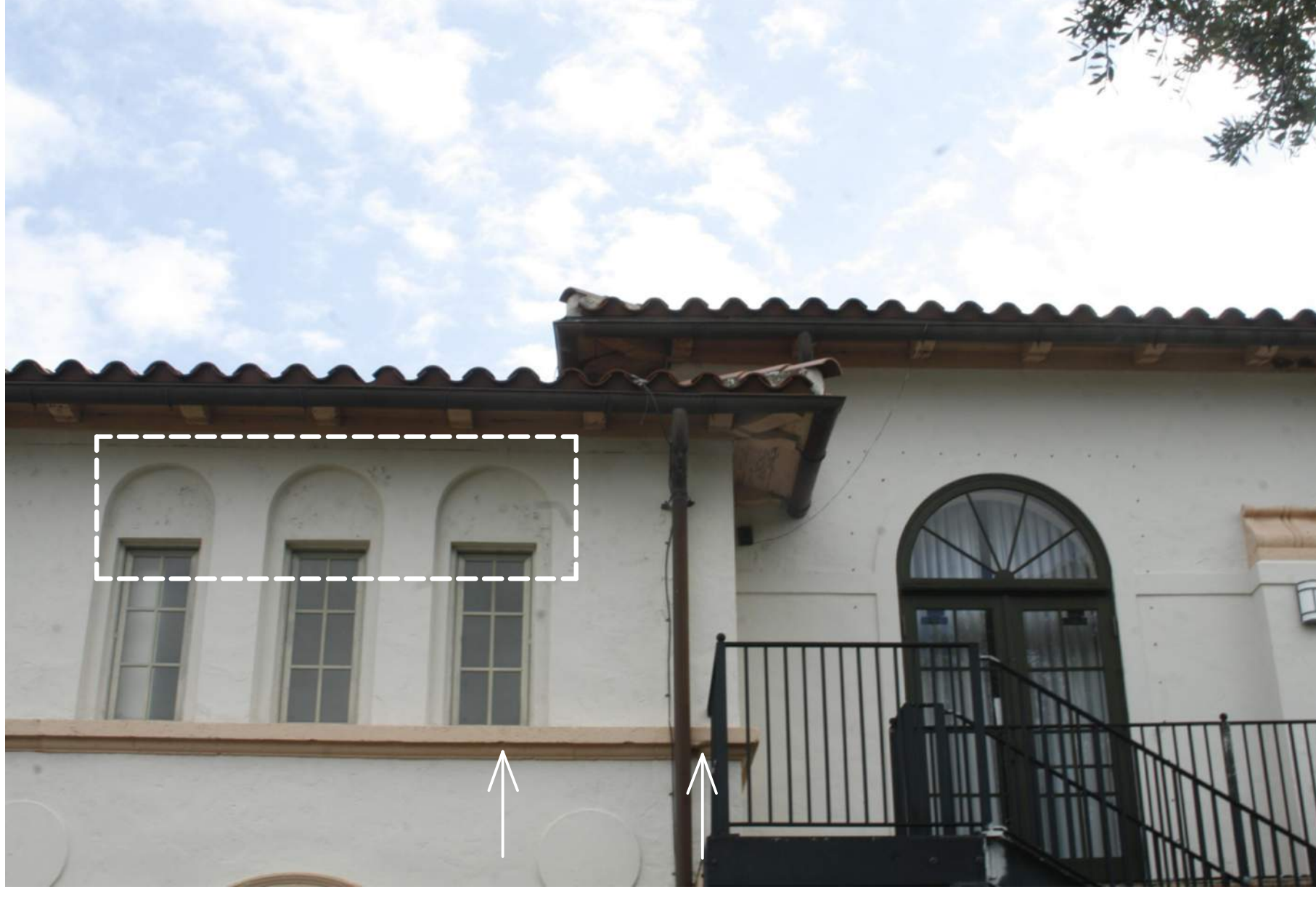
WEST ELEVATION: VERIFY CONDITION OF MOLDING. DETERIORATED STUCCO OR PAINT COAT. V.I.F. IF STUCCO, REFER TO A-23, A-24, A-25 STUCCO FOR STUCCO REPAIS AND COLOR APPLICATION.
