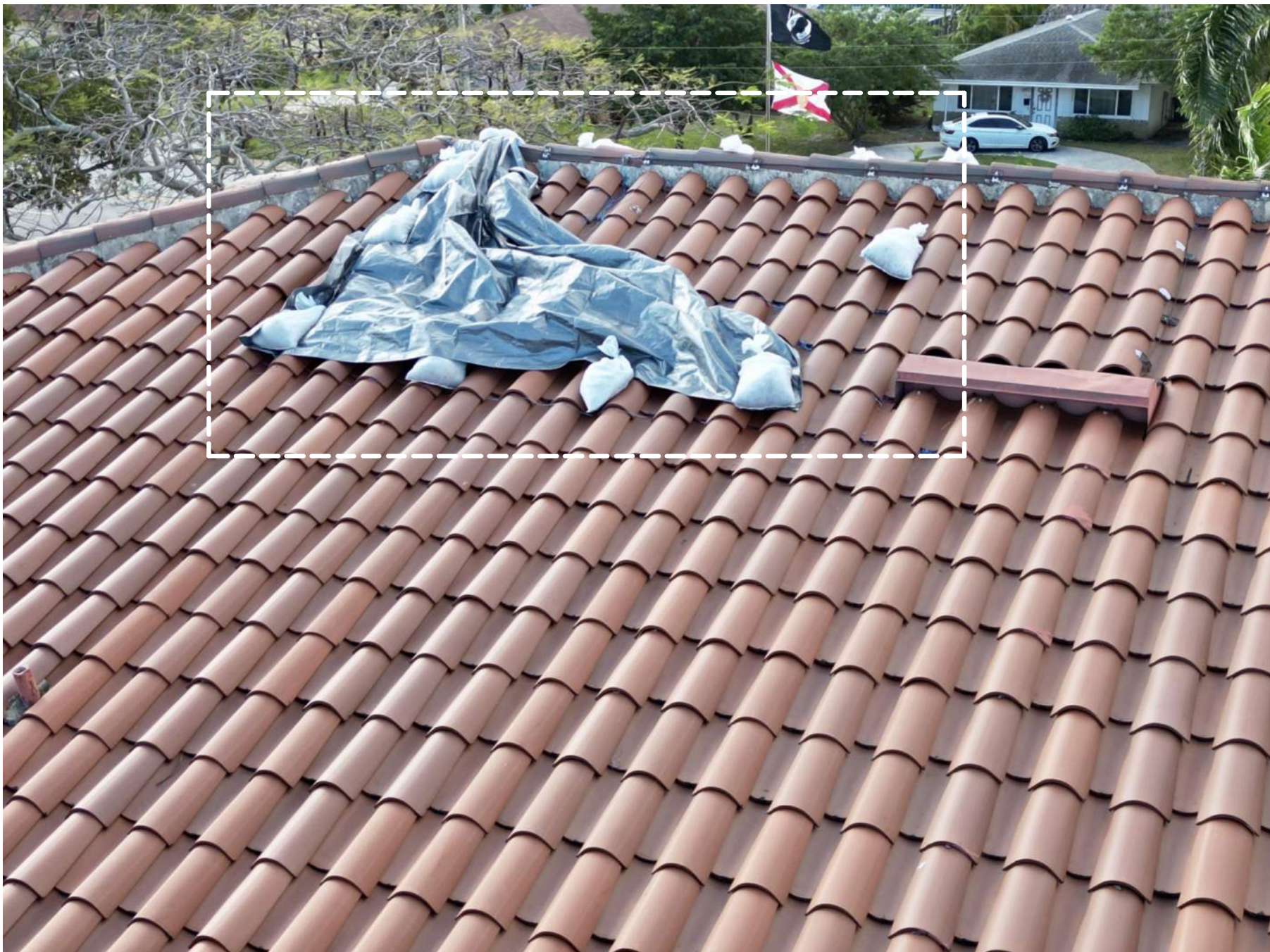
ROOF LEAK SHALL BE REPAIRED
