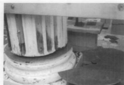
A. This lead sheet was installed at the base of the replacement column to stop rising damp. Photo: Bryan Blumfeld.
