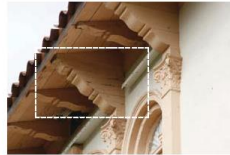
SOUTH ELEVATION: ASSESS DETERIORATION OF PAINT COAT ON RAFTER TAILS AND REPAIR AS NECESSARY.
