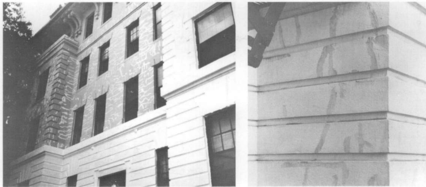
Fig. 13. (a) In preparation for repainting, hairline cracks on this Mediterranean style stucco apartment building were filled with a commercial caulking compound; (b) dirt is attracted and adheres to the texture of the caulked areas, and a year after painting, these inappropriate repairs are highly obvious. Photos: Anne Grimmer.
