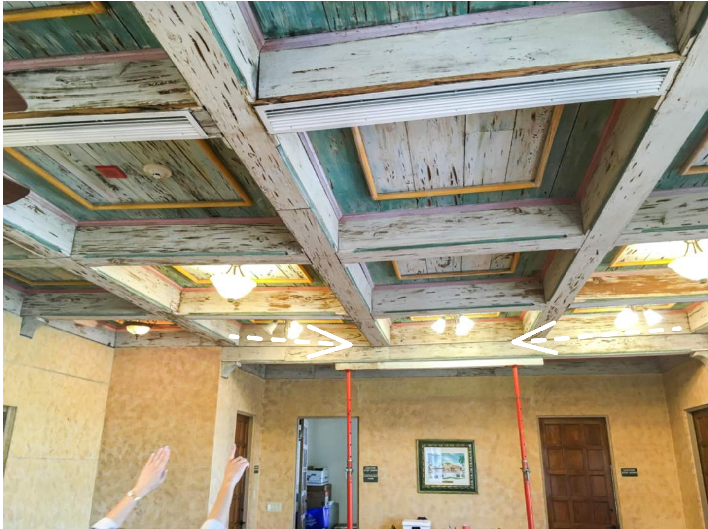
1 DETERIORATED COFFERED CEILING COMPONENTS; SAGGING. REFFER TO SR-1, SR-2, SR-3, SR-4 STRUCTURAL REPORT.
