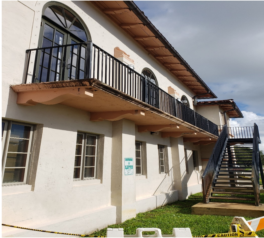
EAST SIDE BALCONY with CONCRETE CANTILEVERED SUPPORT BEAMS
