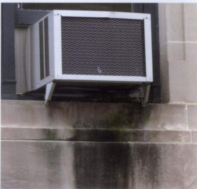
Figure 13. Window air conditioning units can cause damage to surfaces below when condensation drips in an uncontrolled manner. Drip extension tubes can sometimes be added to direct the discharge.
