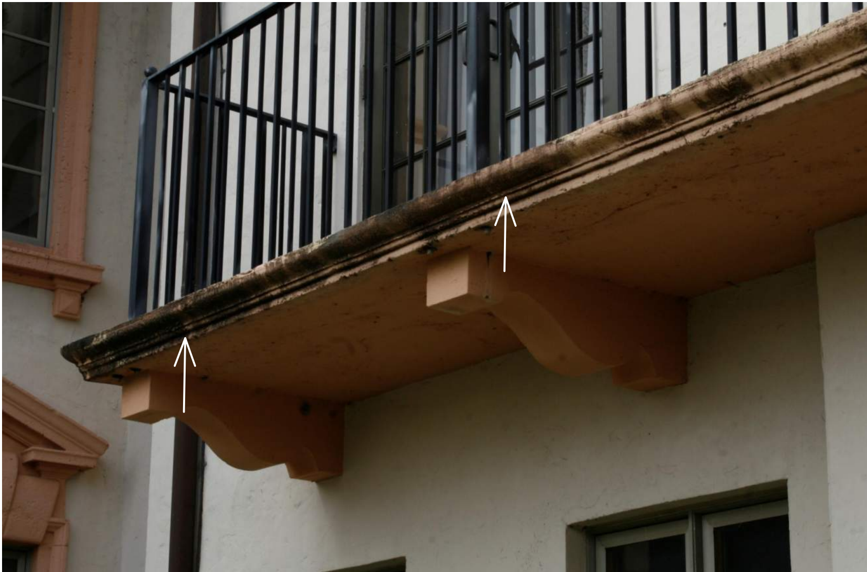
5 EAST ELEVATION: BUILT-UP OF MOLD ON BALCONY SLABS. REFER TO A-20 EXTERIOR CLEANING. ASSESS STRUCTURAL INTEGRITY OF SLAB. REFER TO S-4 IF DAMAGE IS PRESENT.
