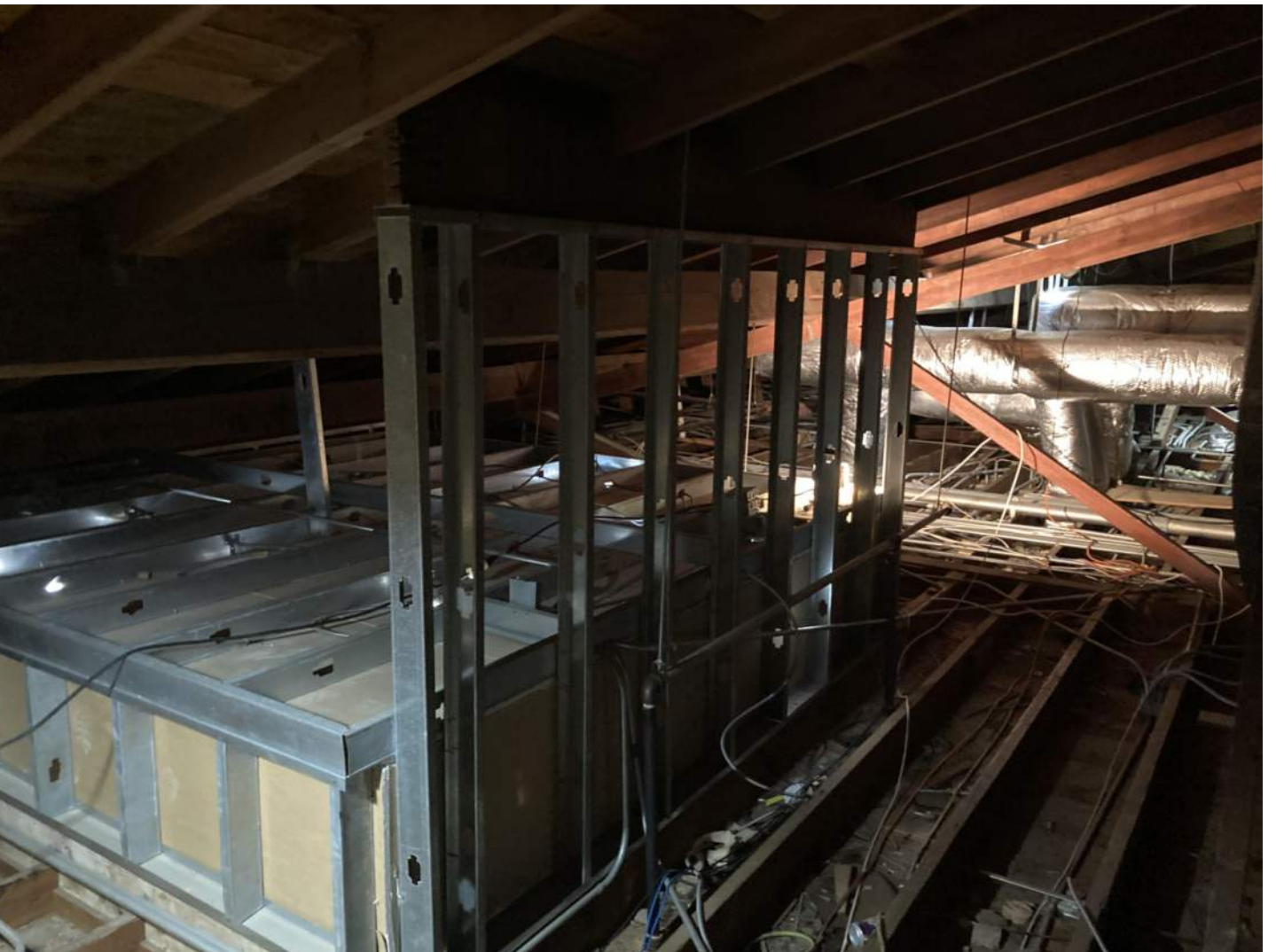
METAL FRAMING SYSTEM UNDER ROOF
