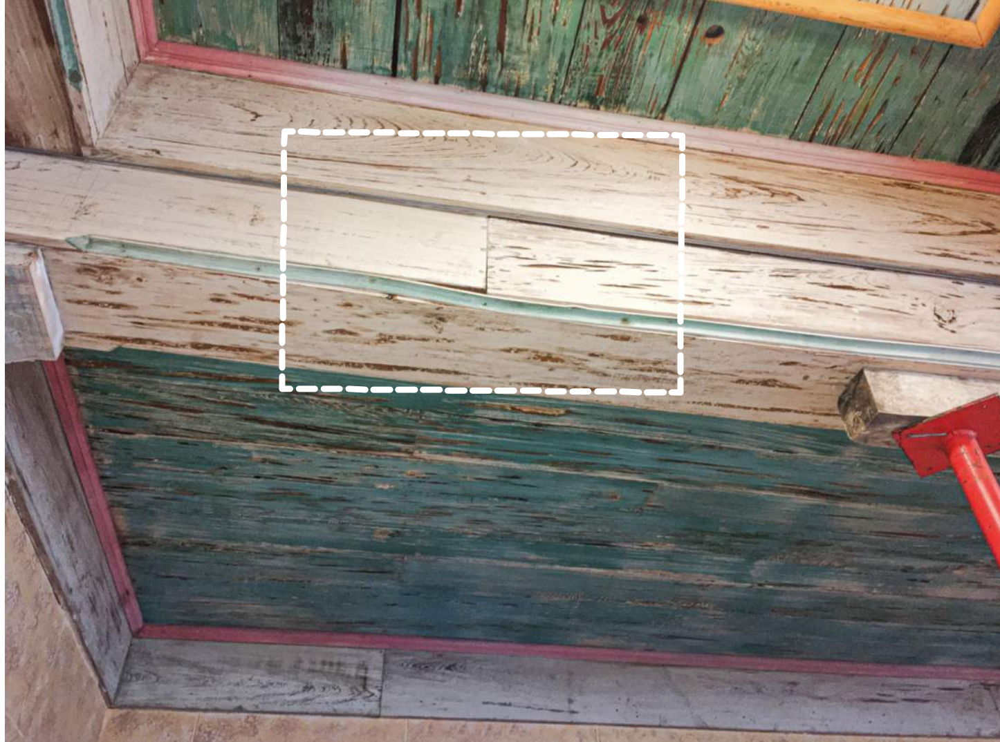
3 DETERIORATED COFFERED CEILING COMPONENTS; SHIFTING. REFFER TO SR-1, SR-2, SR-3, SR-4 STRUCTURAL REPORT.
