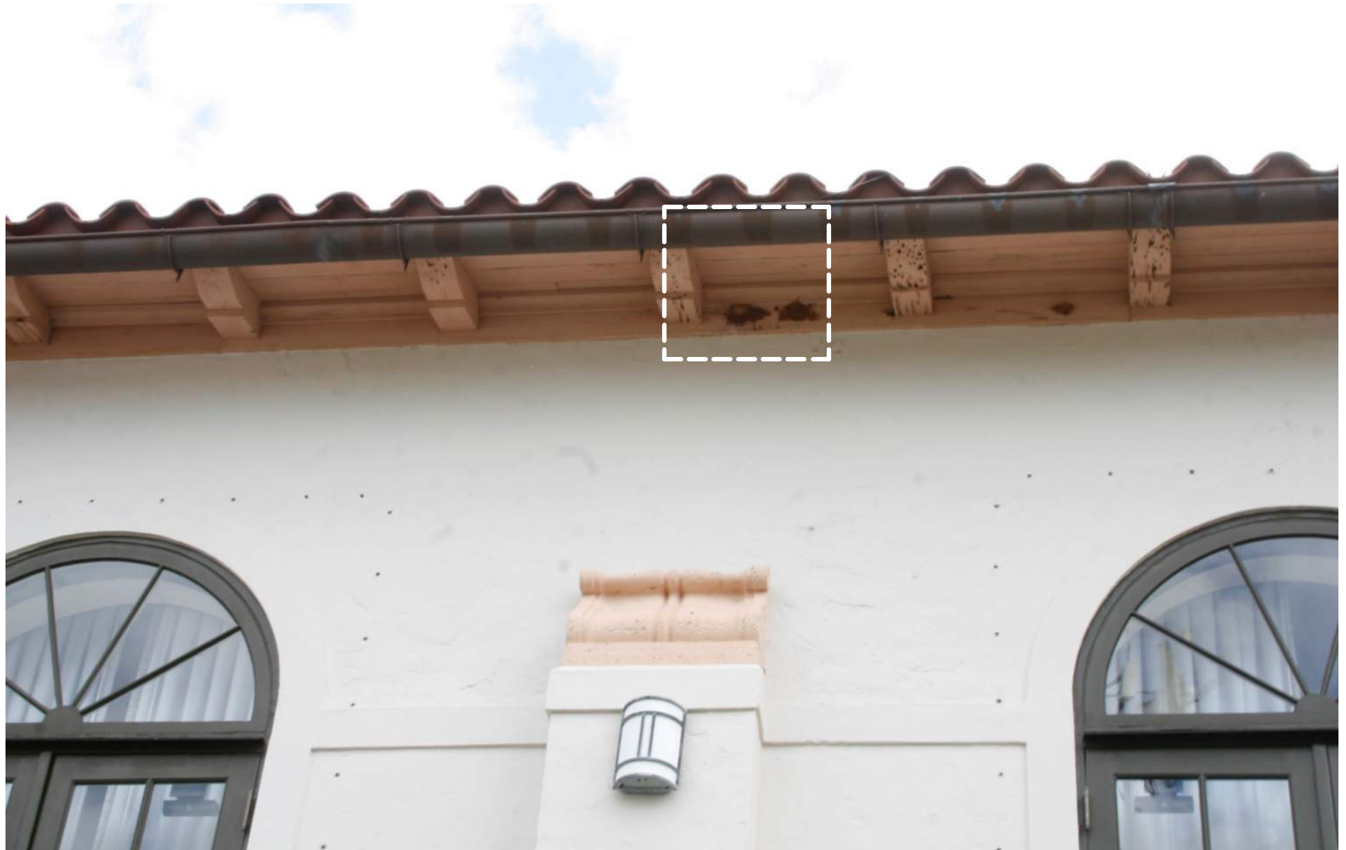
WEST ELEVATION: LOCALIZED CLUSTERS OF UNKNOWN MATERIAL. REFER TO A-20 EXTERIOR CLEANING. V.I.F.
