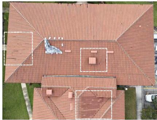
DISCOLORATION OF ROOF TILE, REMOVE ALL VENTS AS REQUIRED.
