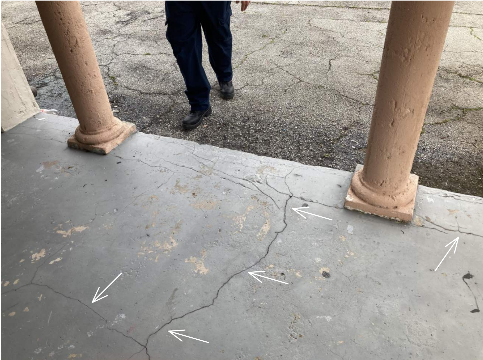
2 NORTH ELEVATION: STRUCTURAL DAMAGE ON FLOOR SLAB. REFER TO S-4 CONCRETE REPAIRS' DETAILS AND PRODUCT SPECIFICATIONS.
