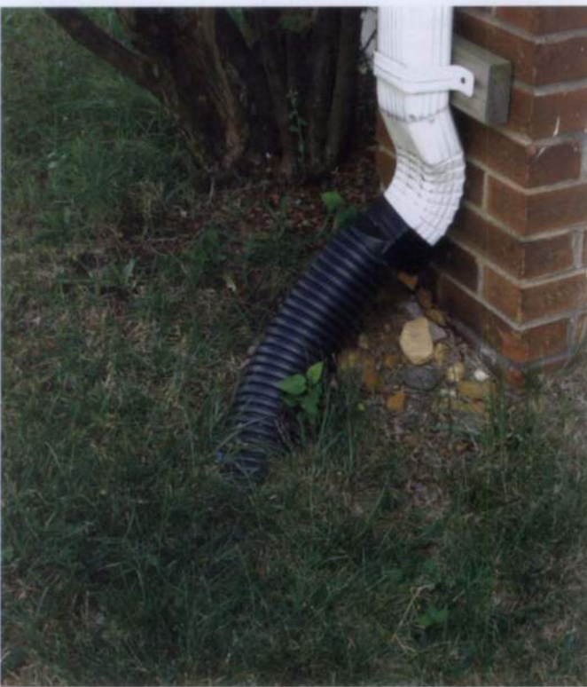
Figure 17. Extending downspouts at their base is one of the basic steps to reduce dampness in basements, crawl spaces and around foundations. Extensions should be buried, if possible, for aesthetics, ease of lawn care, and to avoid creating a tripping hazard.
