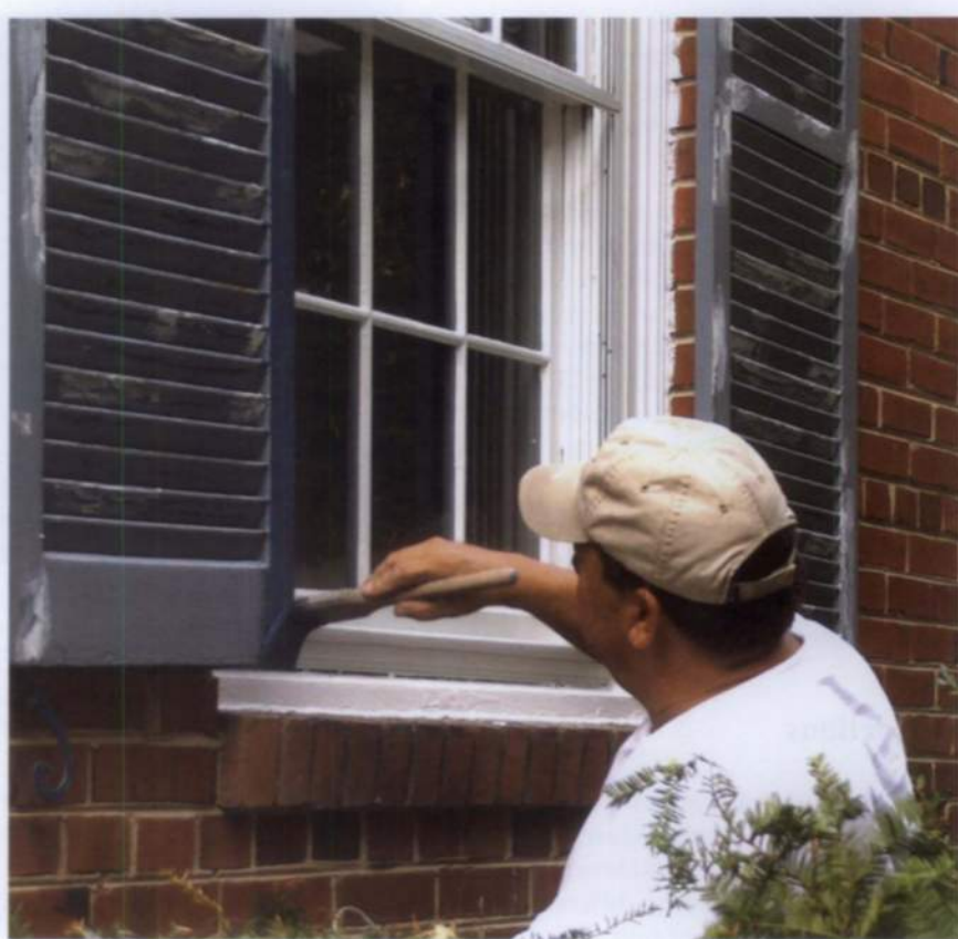
Figure 12. Good surface preparation is essential for long lasting paint. Scraping loose paint, filling nail holes and cracks, sanding, and wiping with a damp cloth prior to repainting are all important steps whether touching up small areas or repainting an entire feature. Always use a manufacturer's best quality paint. Windows and shutters may need repainting every five to seven years, depending on exposure and climate.
