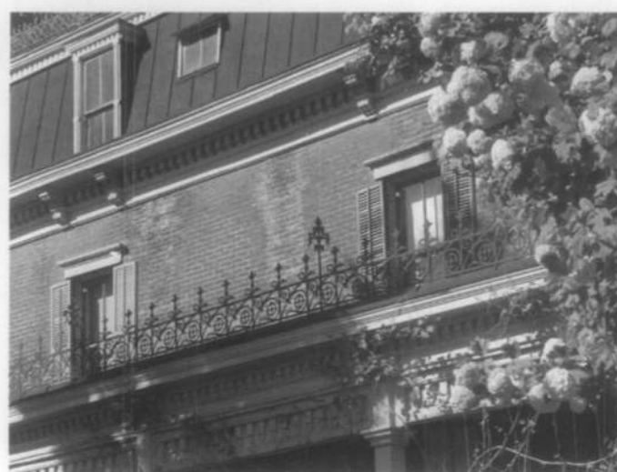
Fig. 4. Deferred maintenance often leads to blocked gutters and downspouts. This cracked gutter system allowed moisture to penetrate the upper exterior wall, erode mortar joints, and rot fascia boards. Photo: NPS Files.
