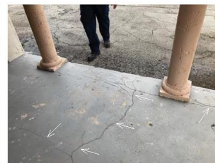
② NORTH ELEVATION: STRUCTURAL DAMAGE ON FLOOR SLAB. REFER TO S-4 CONCRETE REPAIRS' DETAILS AND PRODUCT SPECIFICATIONS.
