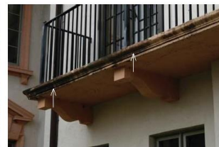
⑤ EAST ELEVATION: BUILT-UP OF MOLD ON BALCONY SLABS. REFER TO A-20 EXTERIOR CLEANING. ASSESS STRUCTURAL INTEGRITY OF SLAB. REFER TO S-4 IF DAMAGE IS PRESENT.
