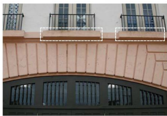
NORTH ELEVATION: FACADE DISCOLORATION. V.I.F.
