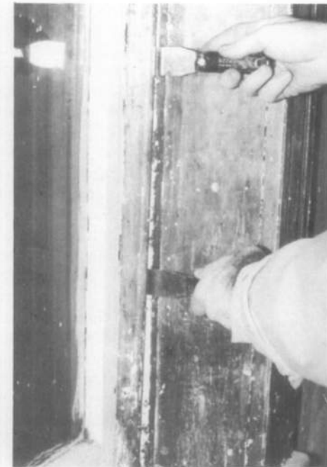
Figure 4b. After removing paint from the seam between the interior stop and the jamb, the stop can be pried out and gradually worked loose using a pair of putty knives as shown. To avoid visible scarring of the wood, the sash can be raised and the stop pried loose initially from the outer side. Photo: John H. Myers
