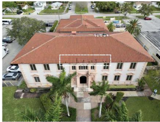
MAIN ENTRANCE SOUTH AERIAL VIEW ROOF CONDITION, MISSING ROOF TILES
