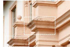
SOUTH ELEVATION: BUILD-UP OF MOLD ON LEGDE SURFACE. REFER TO A-20 EXTERIOR CLEANING.
