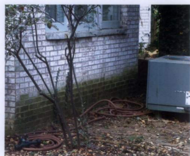
Figure 17. This chronically wet area has a mildew bloom brought on by heat generated from the air-conditioning condenser unit. The dampness could be caused by a clogged roof gutter, improper grading, or a leaking hose bibb.
