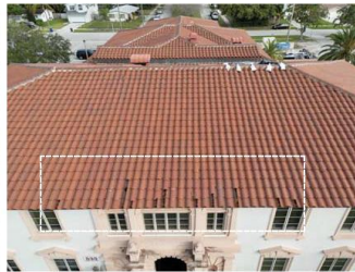
SOUTH AERIAL ROOF VIEW / MISSING AND CHIPPED ROOF TILES, REMOVE ALL VENTS AS REQUIRED
