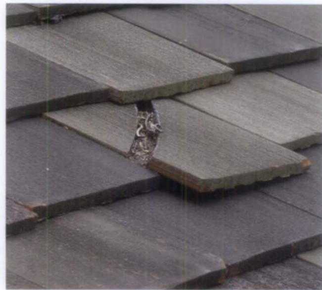
Figure 4. Damage to roofs often requires immediate attention. As a temporary measure, this damaged roof tile could be replaced with a brass aluminum sheet wedged between the existing tiles. Photo: Chad Randall.
