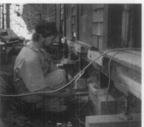
B. Wood sills set on grade were replaced with concrete pier foundation and new wooden sill plates. Changes were not visible on the exterior (see C). Photo: WPTC, NPS.
