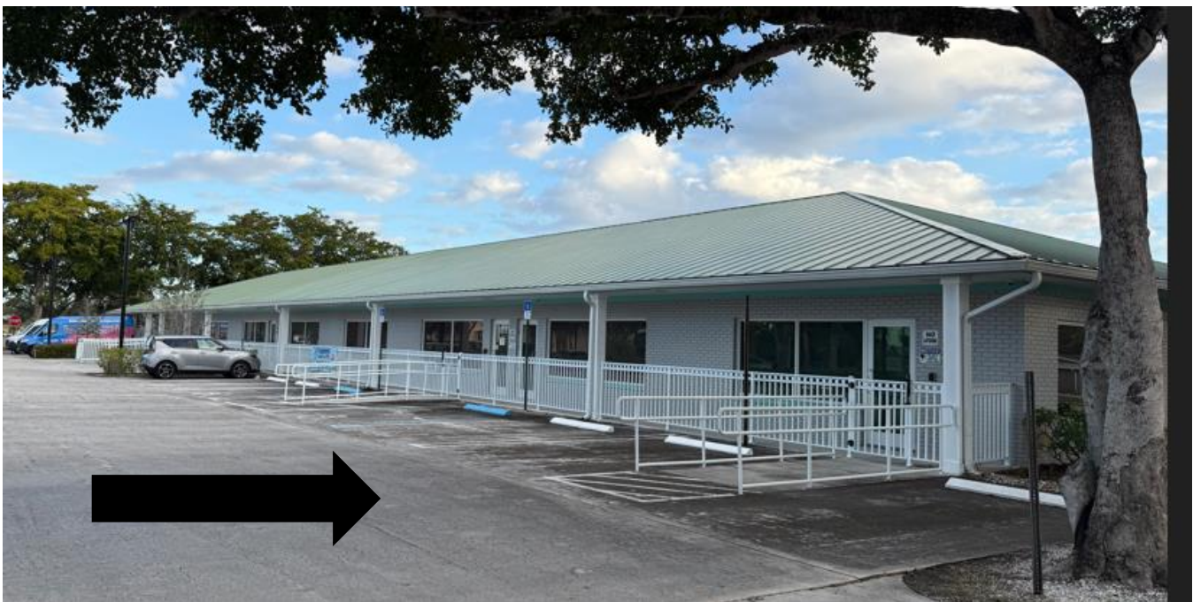
South End of Building – Proposed Location
