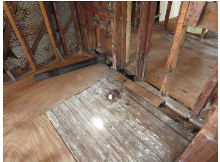
Discontinuous floor deck sheathing PHOTO NO. IMG_8011
