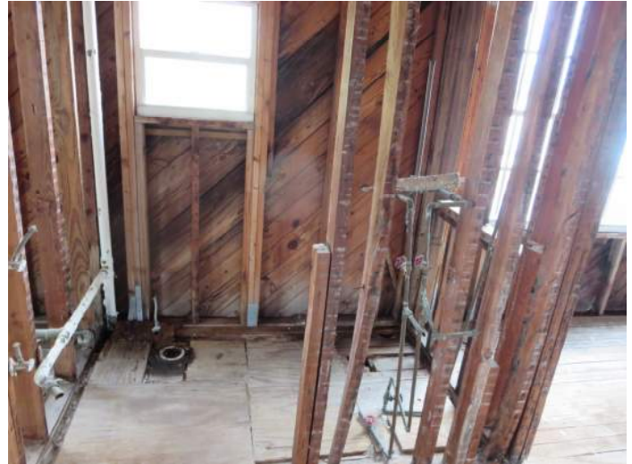
Discontinuous floor deck sheathing PHOTO NO. IMG_8002
