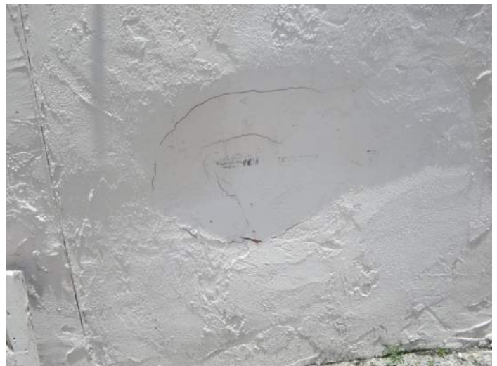
Stucco finish indentation PHOTO NO. IMG_7931
