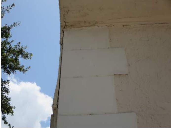
Finish separation PHOTO NO. IMG_7919
