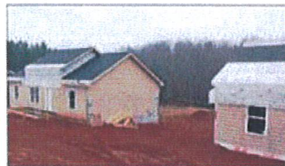
There will eventually be a total of 31 single family homes in the Creekwood Meadows neighborhood in Rutherfordton.
