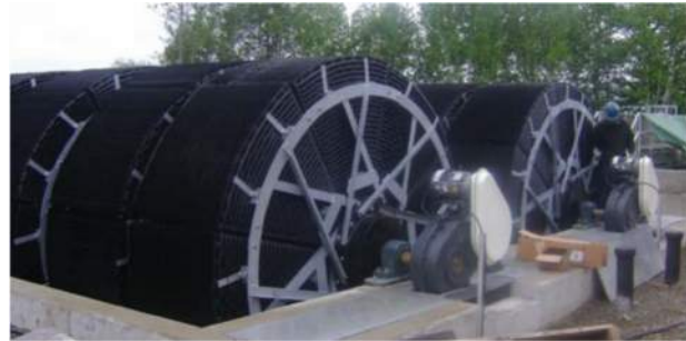
Evoqua Water Technologies Envirex® RBC Units
