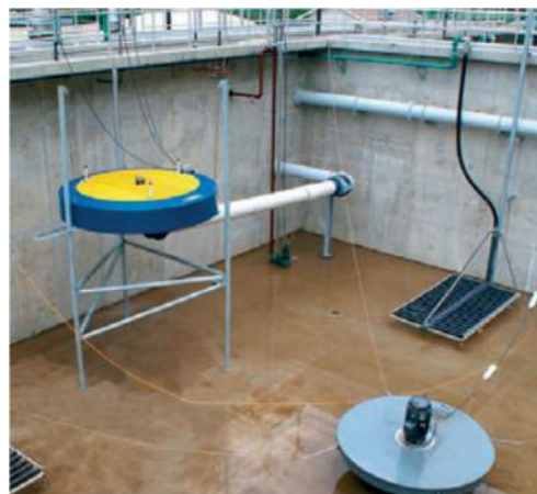
Emptied Alfa Laval AS-H SBR Reactor
