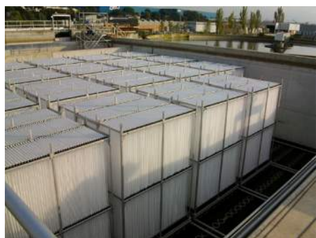
Ovivo Cleartec® IFAS Fixed Media Racks
