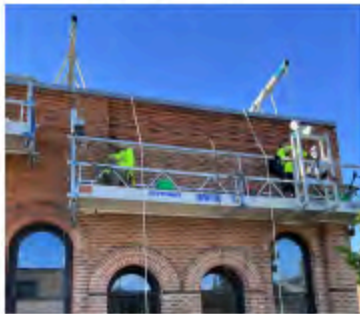
Flashing Installation
