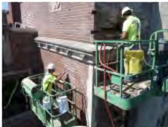
Tuckpointing & Brick Repairs
